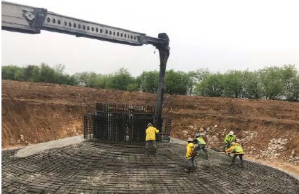
Picture 1. Placing foundation base concrete.
