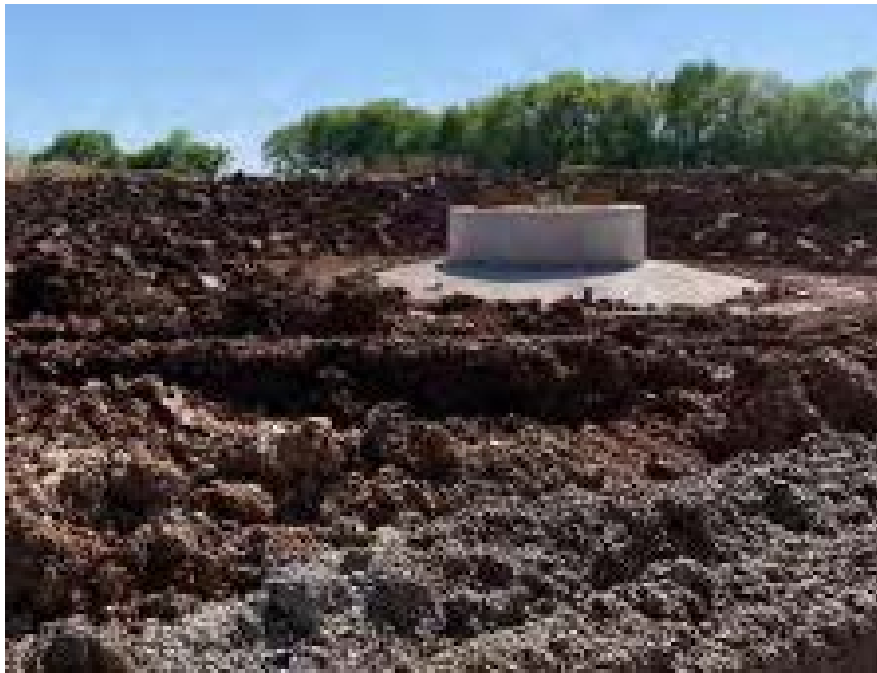
Picture 2. Foundation for T-55 backfilled and compacted.
