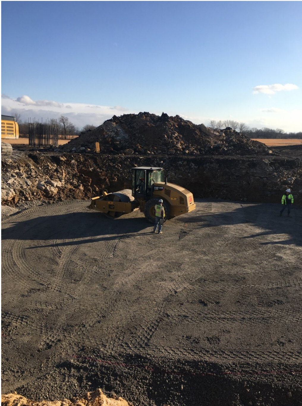
Rolling base of foundation
