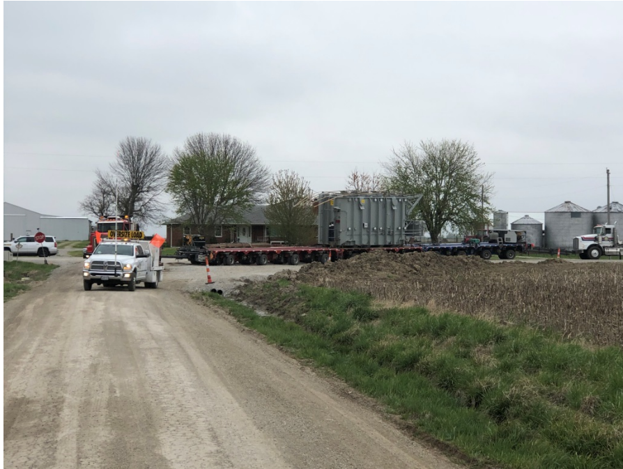
Picture 1. Main power transformer en route from Asbury Plant to project substation site (April 3, 2020).
