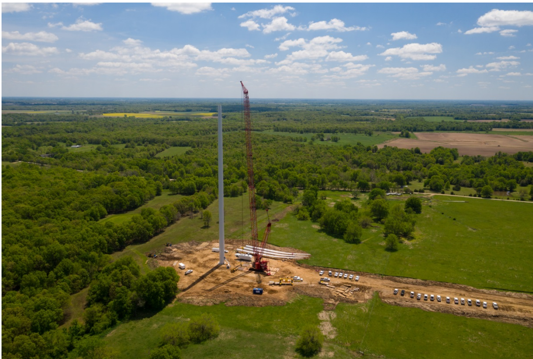
Picture 4. Erecting tower for T-94 (April 30, 2020).
