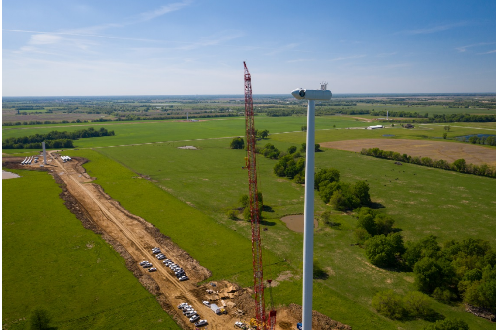
Picture 5. Nacelle in place on T-94 (April 30, 2020).
