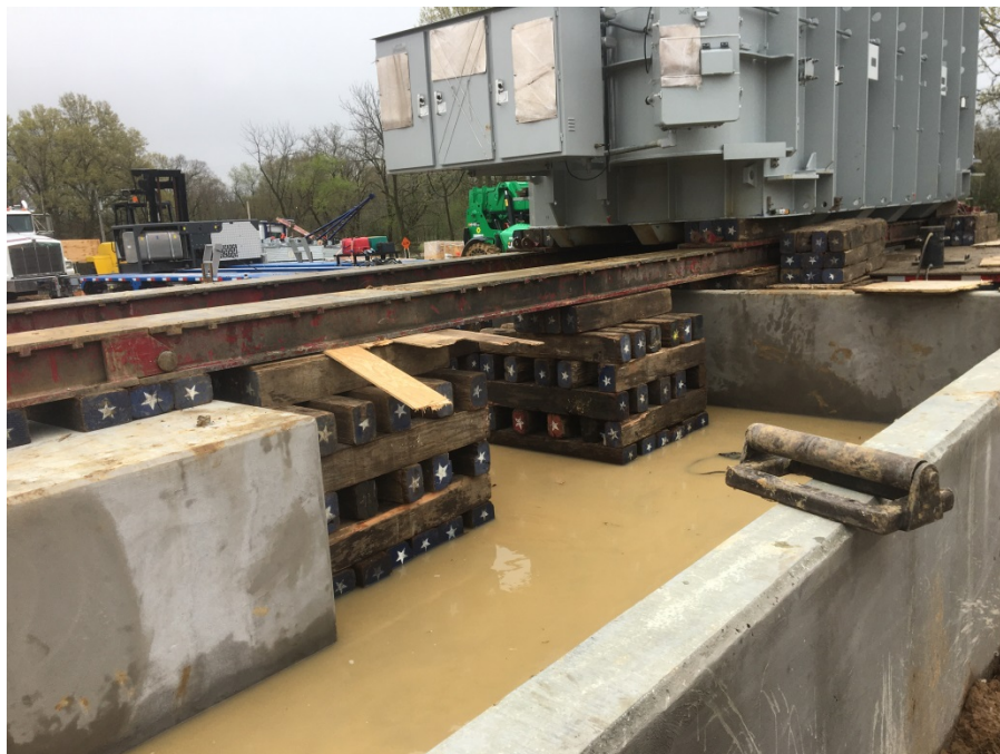
Picture 2. Main transformer being moved from trailer to foundation (April 4, 2020).
