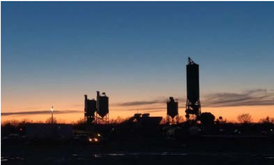
Picture 4. Concrete batch plant.
