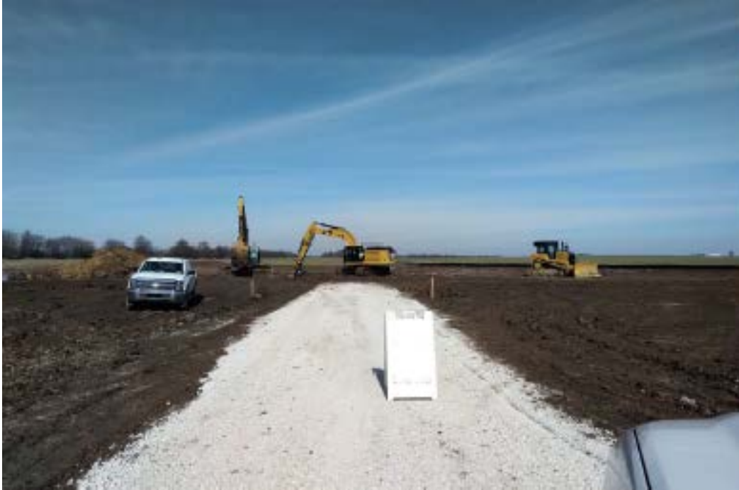
Picture 3. Foundation excavation.
