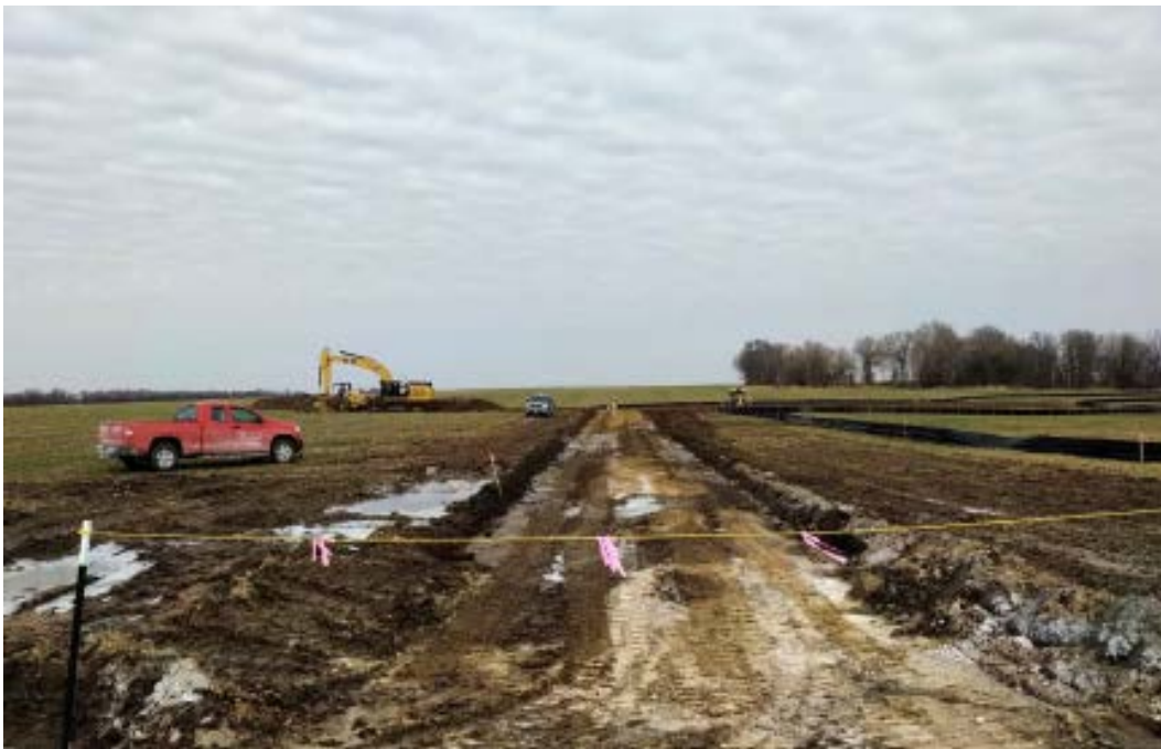
Picture 2. Stabilized access road.
