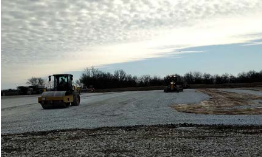
Picture 1. Laydown yard installation.
