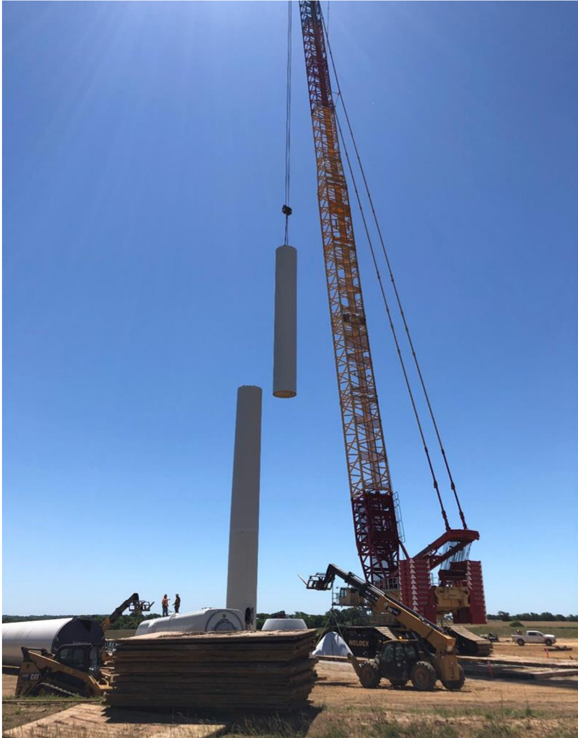
Tower Section Installation
