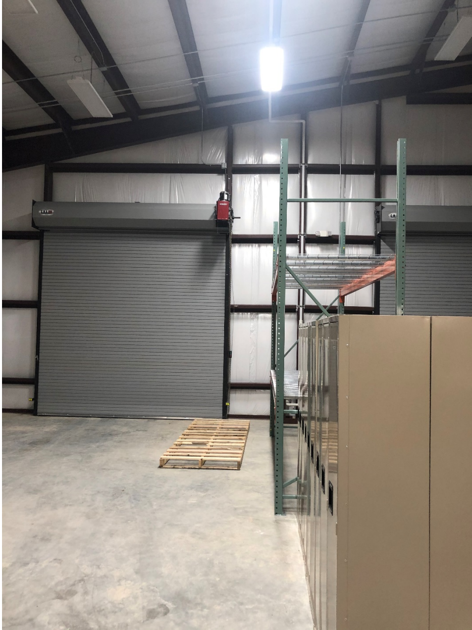
O&M Building – Shop Area
