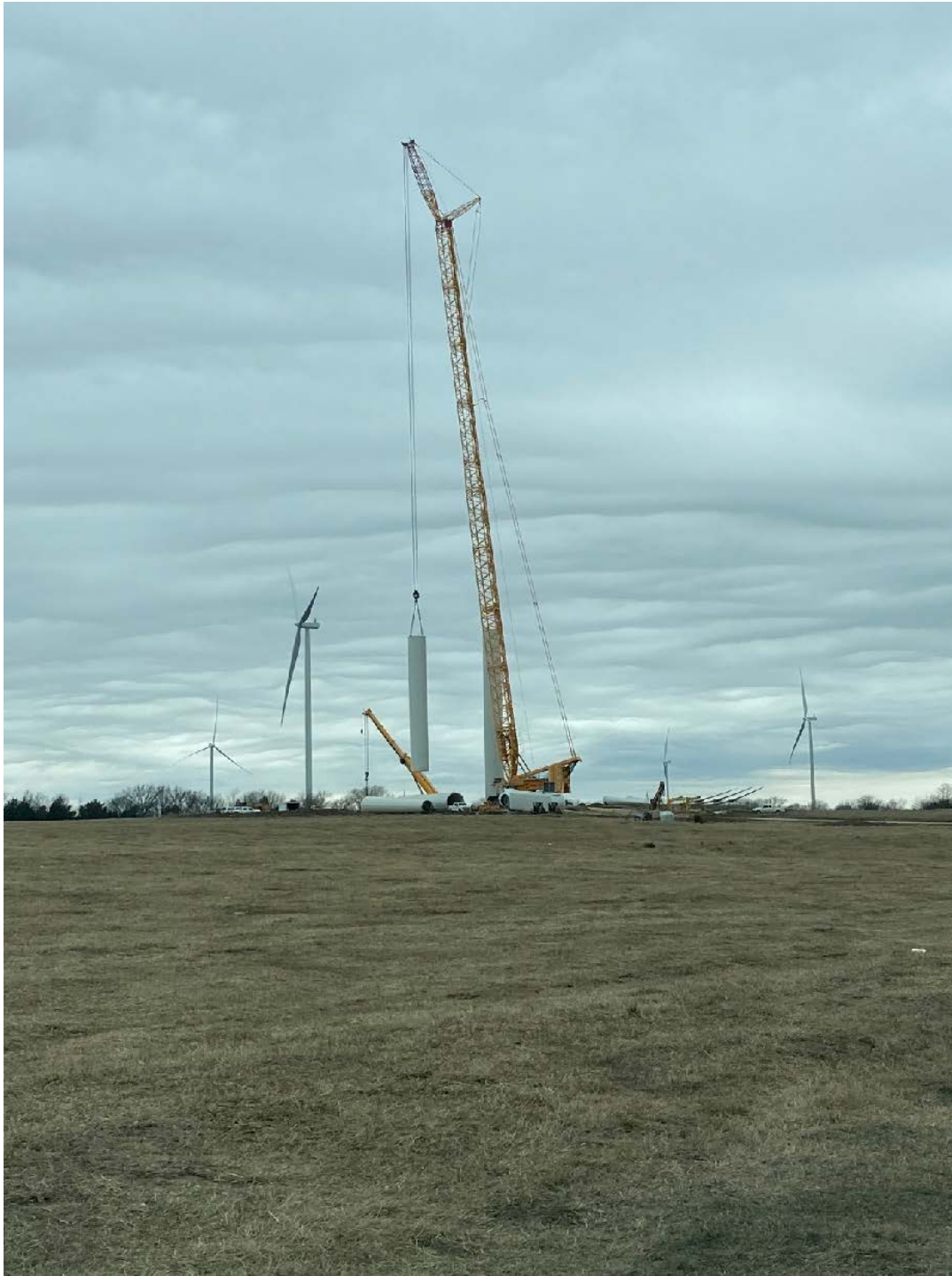
Tower Section Installation
