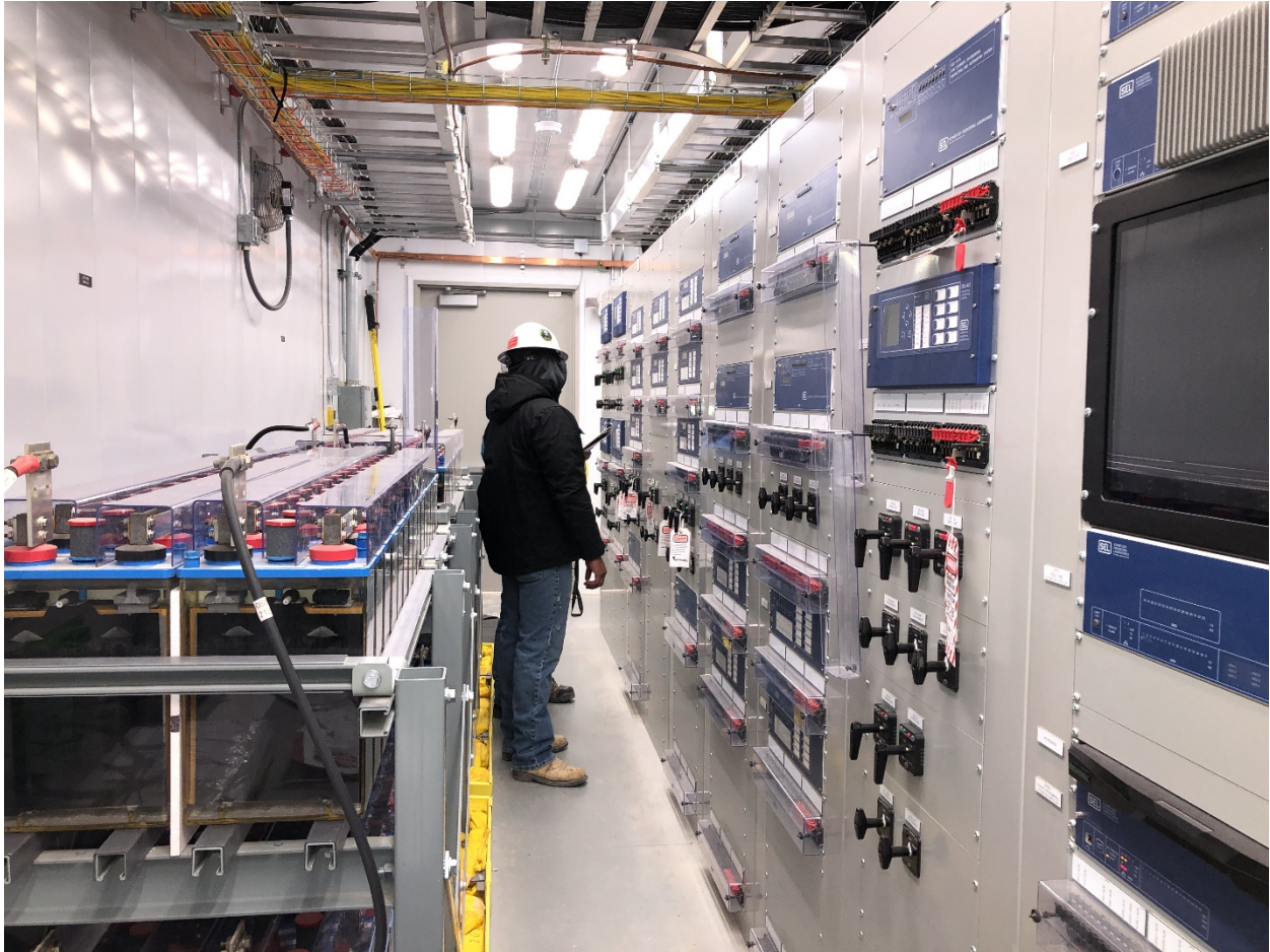
Control Building Interior
