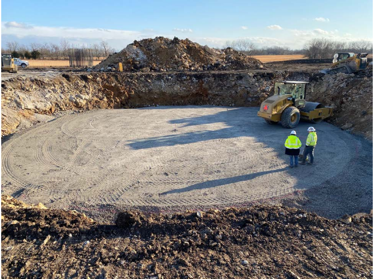
Prepping foundation for mud mat
