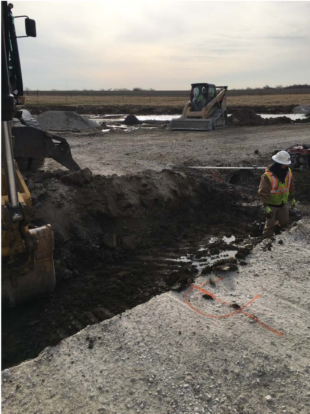
Substation foundation preparation
