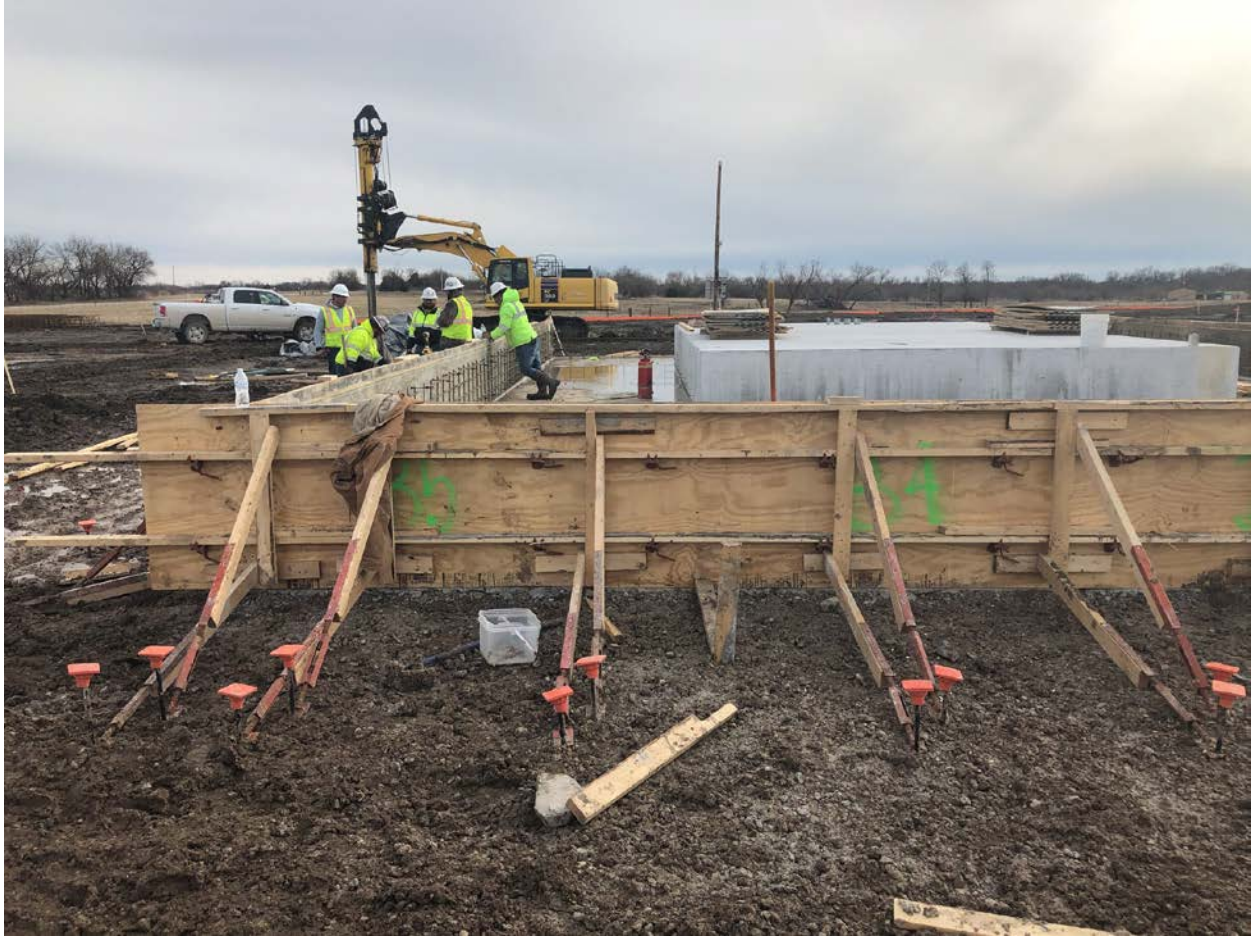
Forming of containment wall of Main Power Transformer
