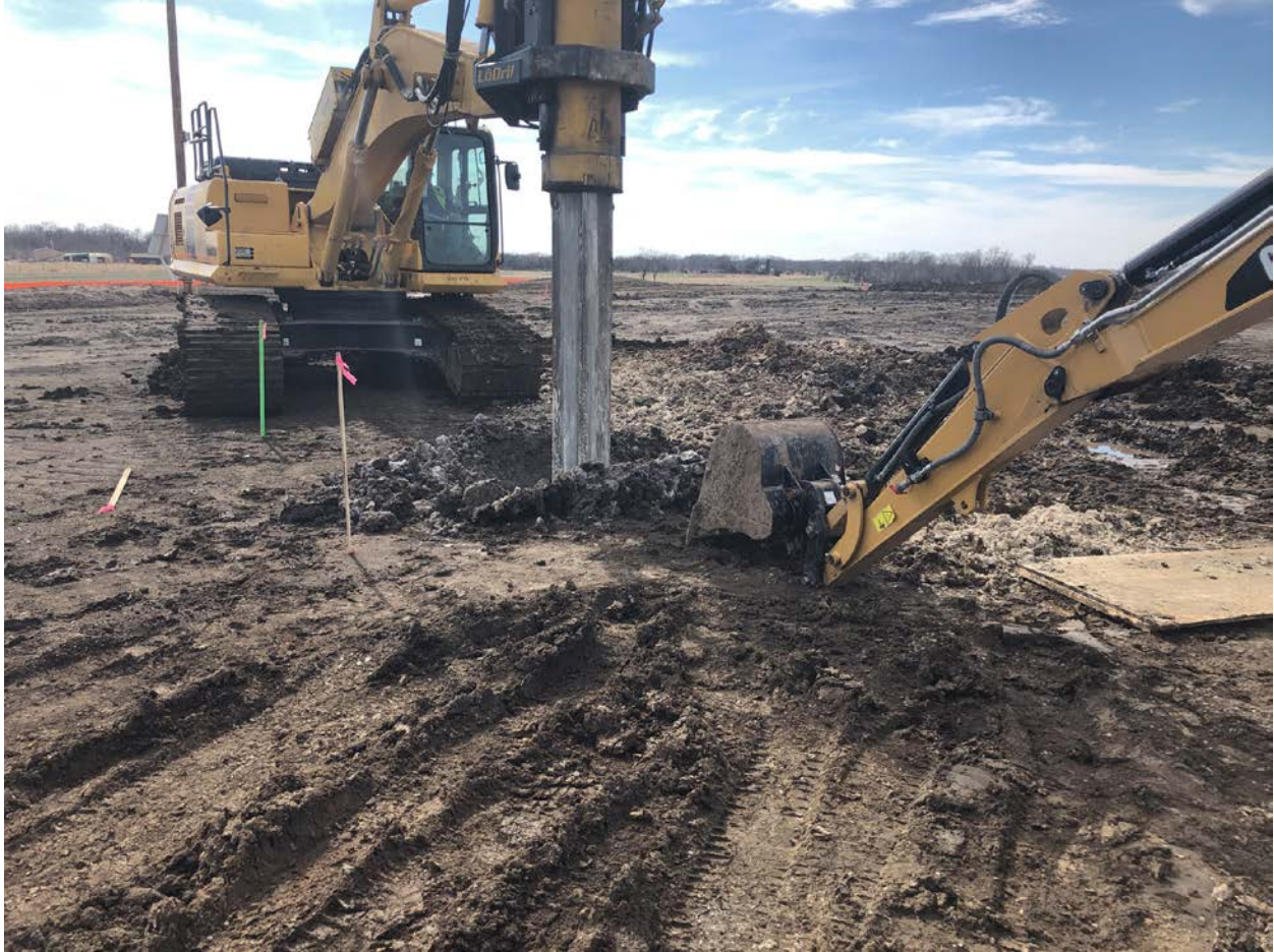
Drilling pier foundation for control room
