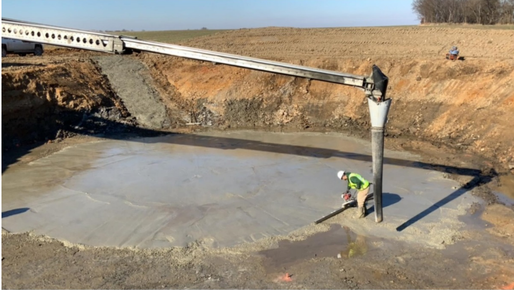
Picture 1. Using a telebelt to place mud mat.
