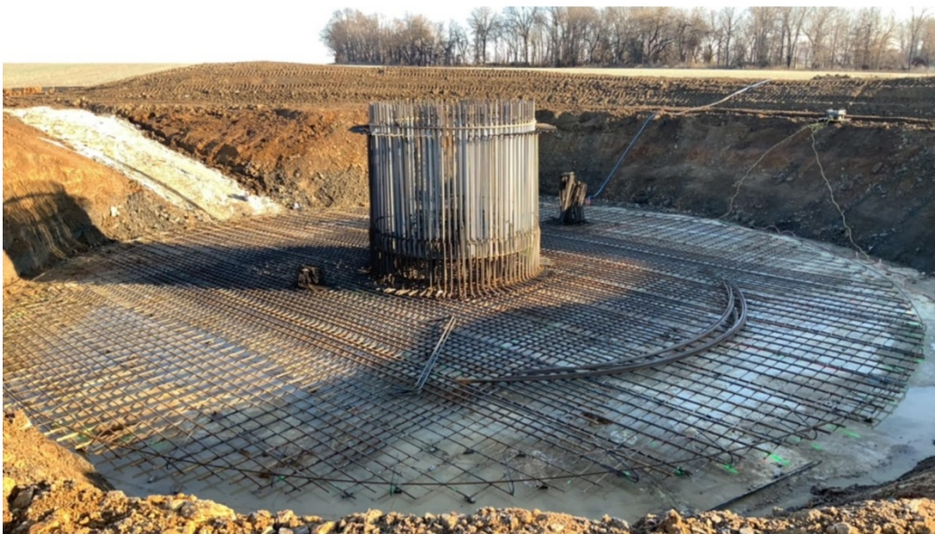
Picture 2. Bottom rebar mat and anchor bolt cage.
