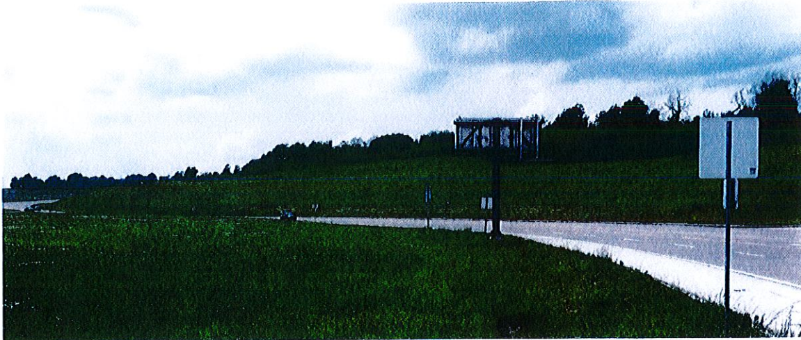
Project Site Looking West from Missouri Bottom/N. Lindbergh Intersection
