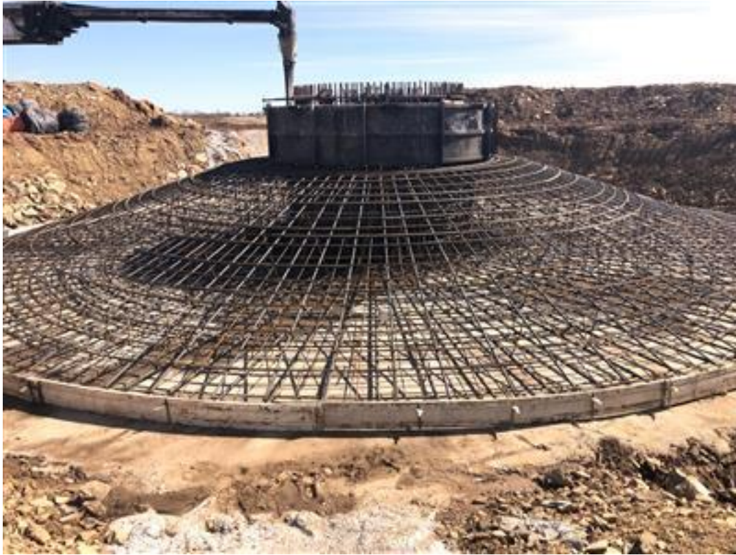
Foundation Rebar
