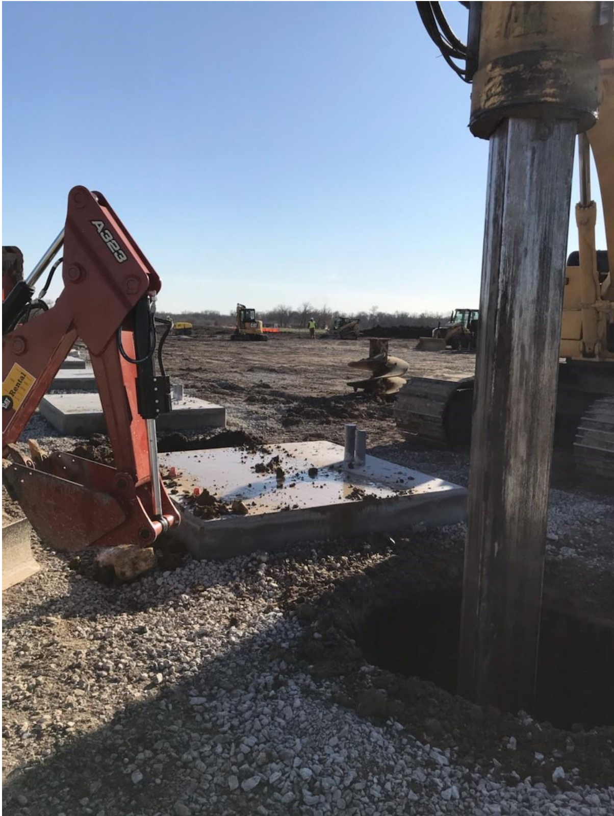
Substation Flatwork Foundation
