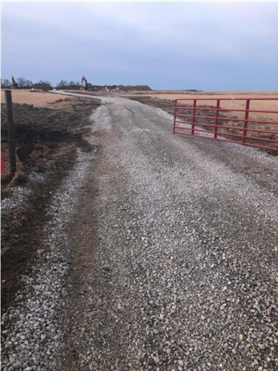
Completed Access Road
