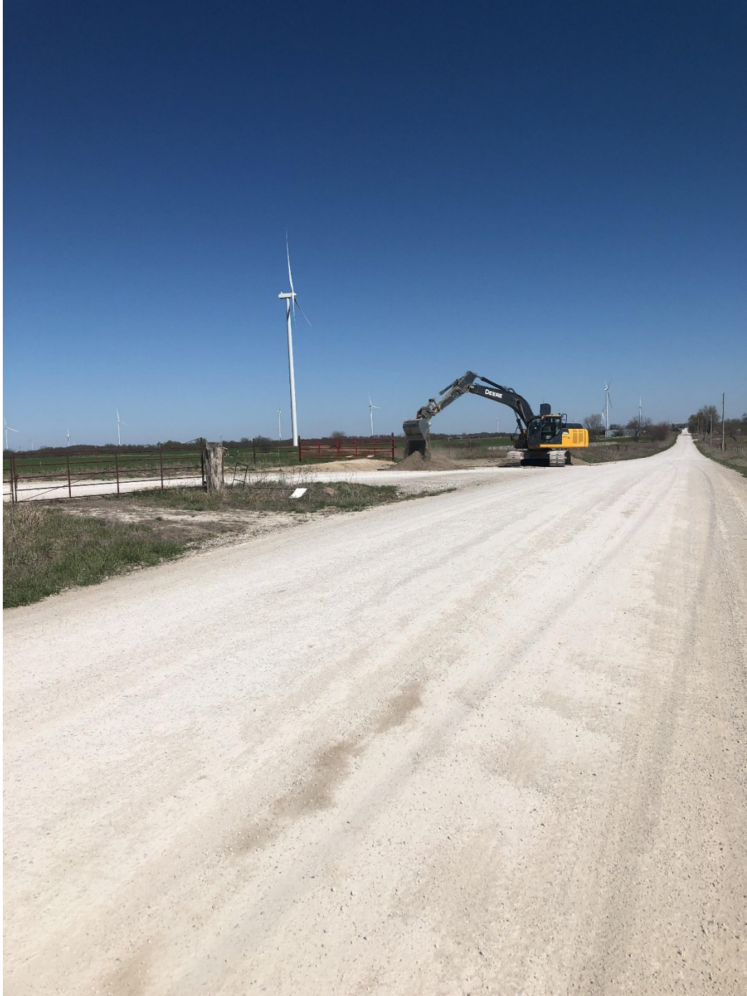
Public Road Restoration
