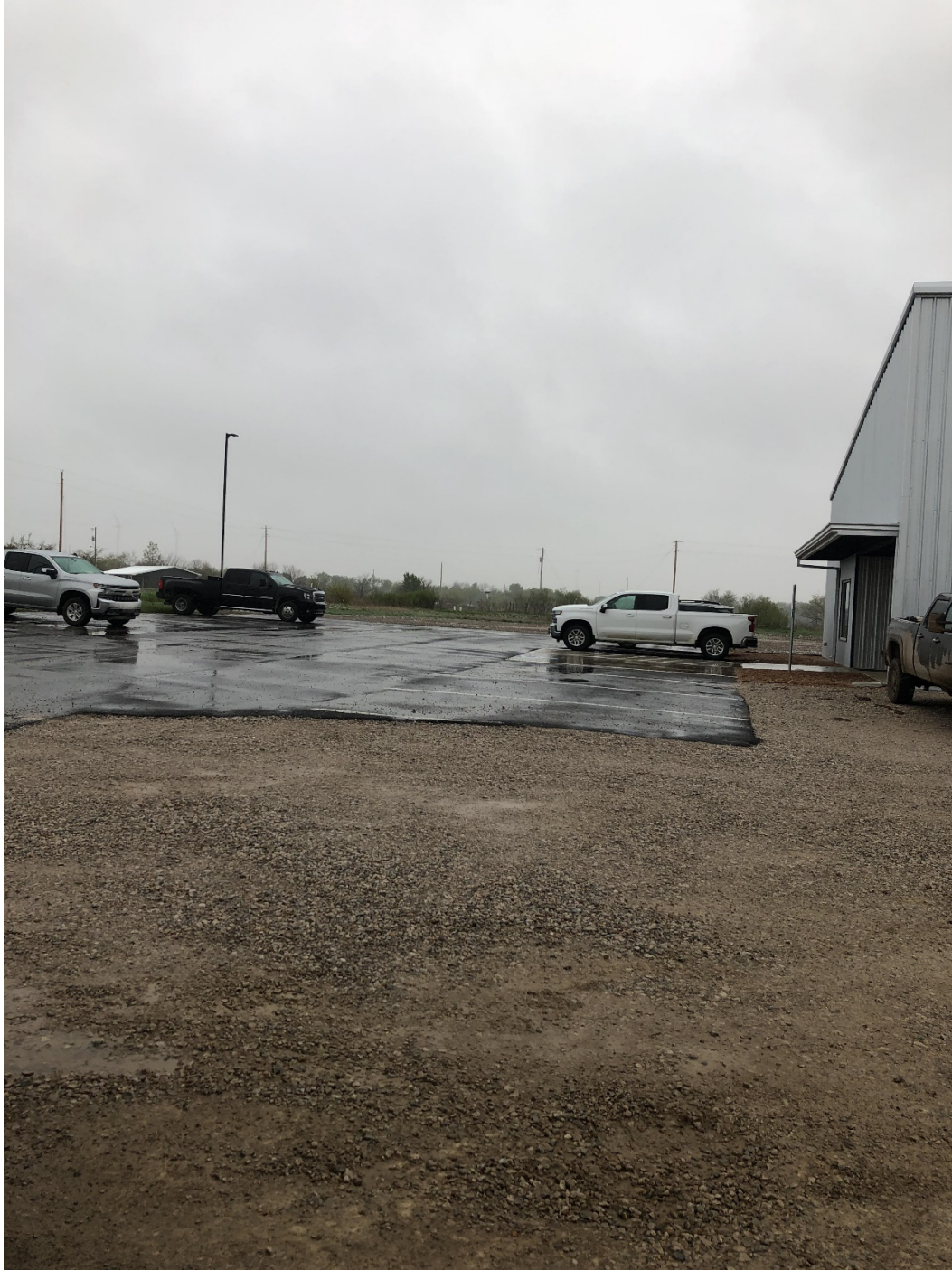
O&M Building Exterior and Parking Lot
