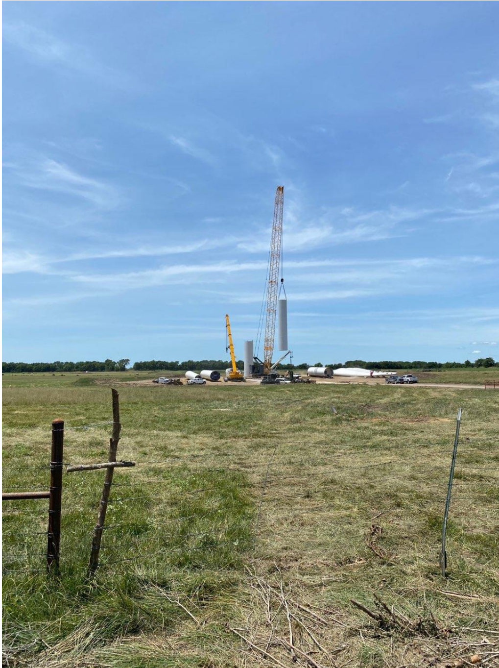
Tower Section Install
