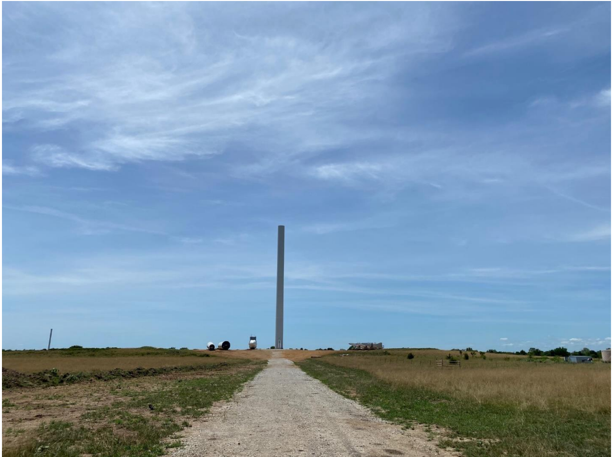
Tower Sections and Access Road
