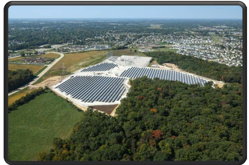
O'Fallon Renewable Energy Center. Missouri's largest investor-owned utility solar facility, and contains over 19,000 solar panels.
