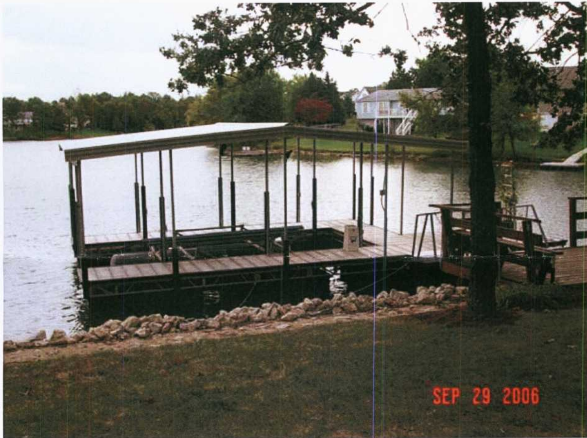
Photo of the dock where the accident occurred.
