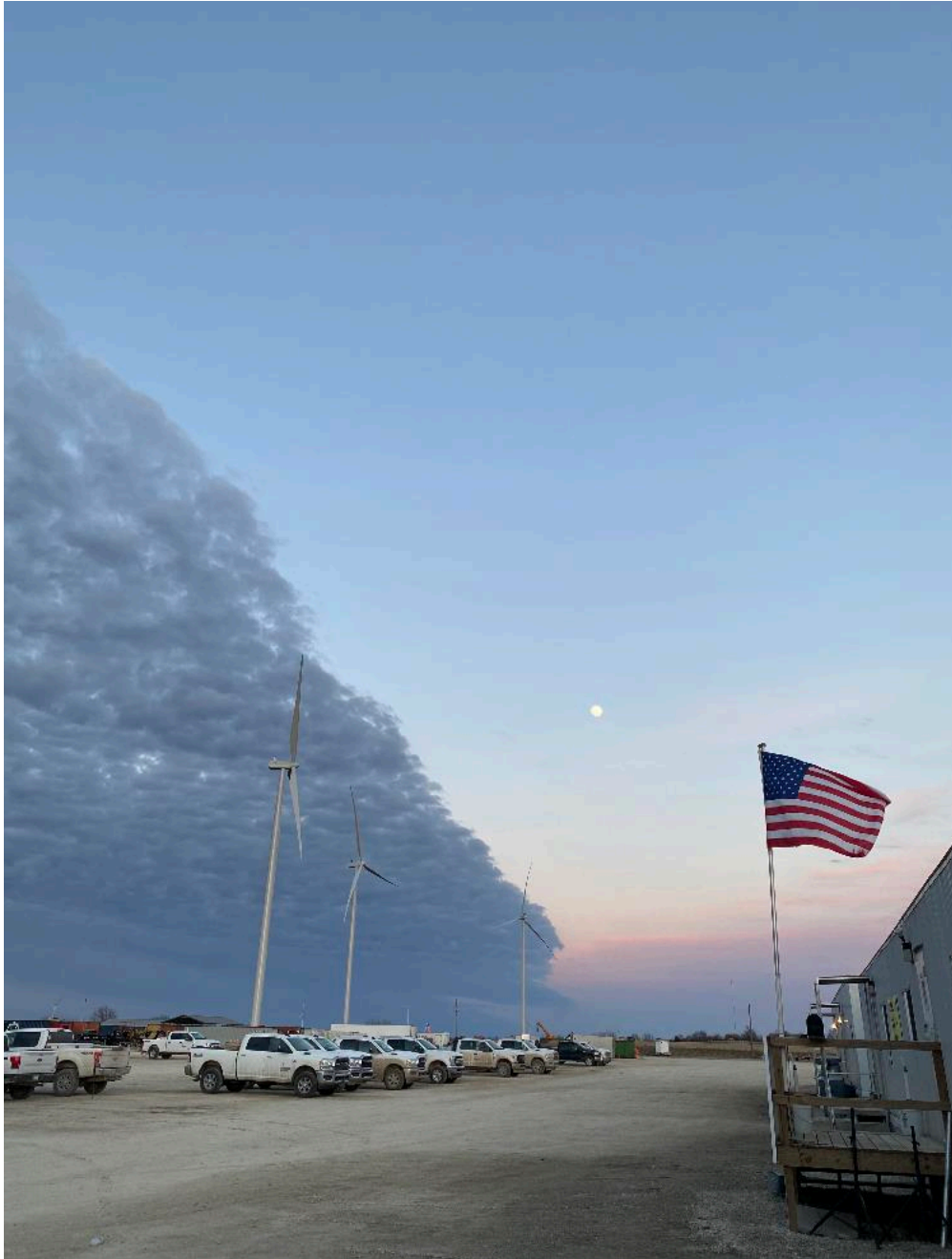
View of Turbines from Laydown Yard
