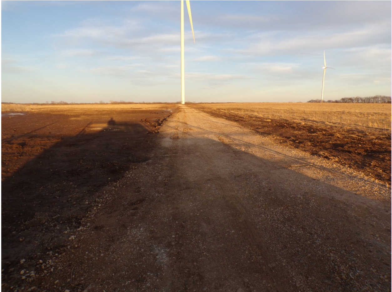
Access Road and Base of Turbine
