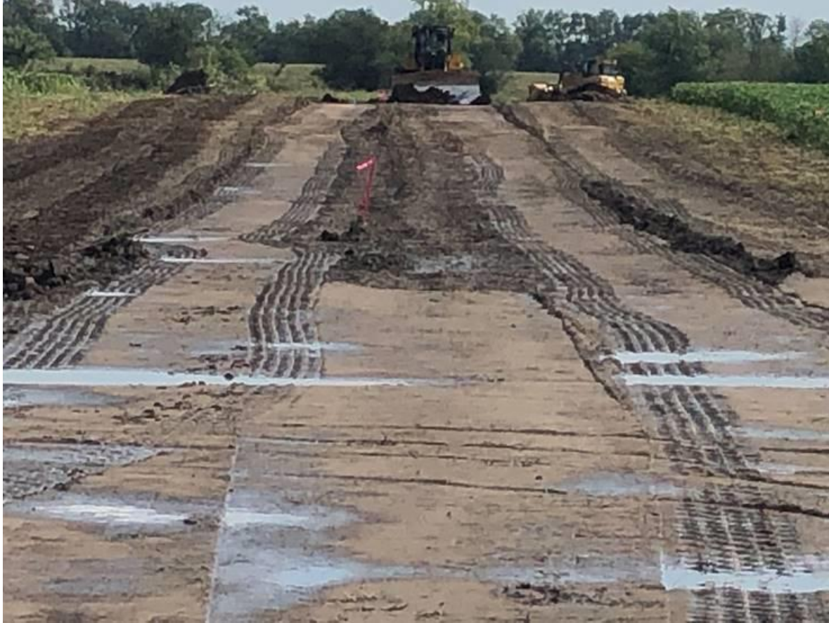
Stripping Access Road
