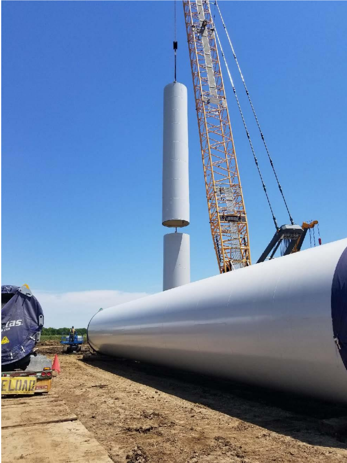
Turbine Erection
