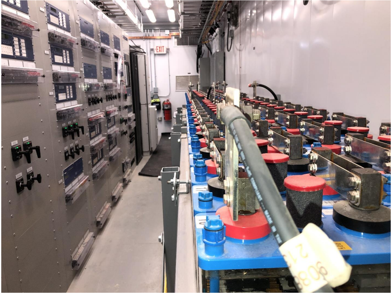
Control Building (Interior)
