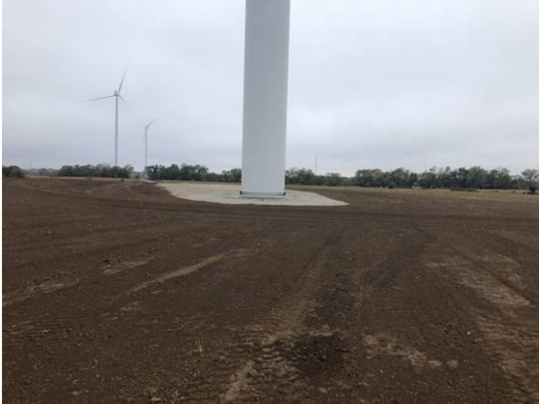
Turbine Site Restoration
