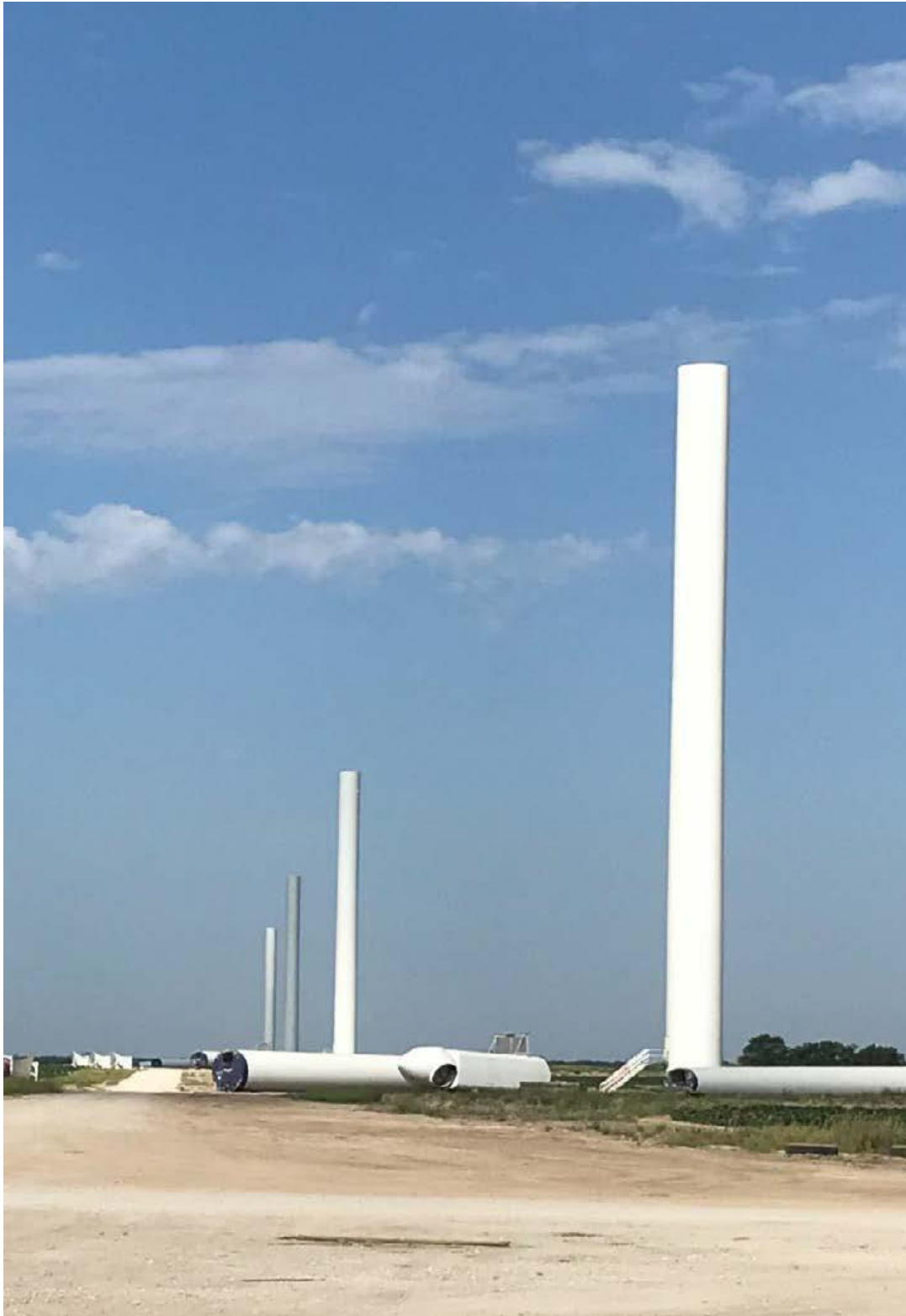
Installed Tower Sections with Stage Turbine Components
