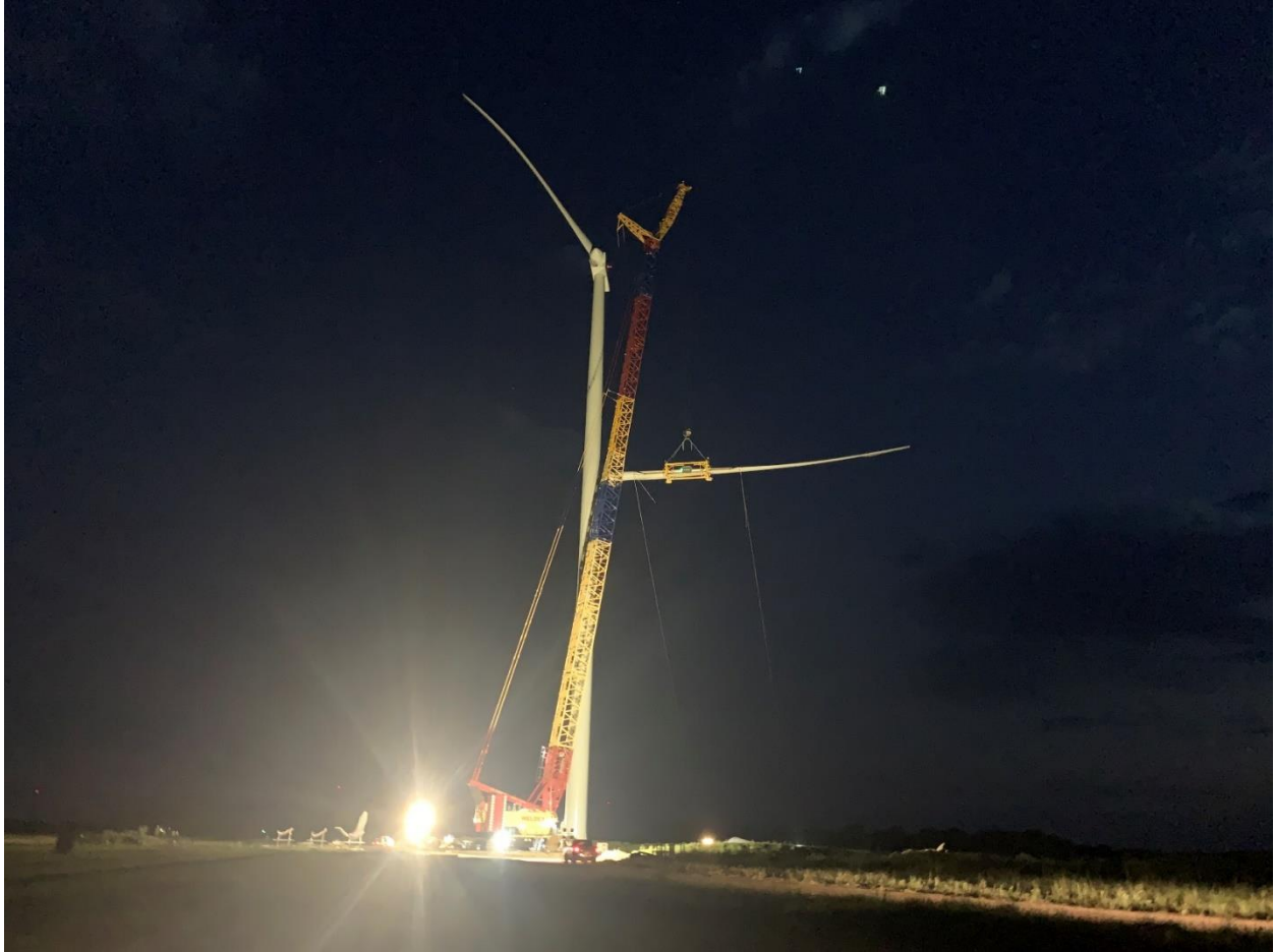
Blade Install at Night
