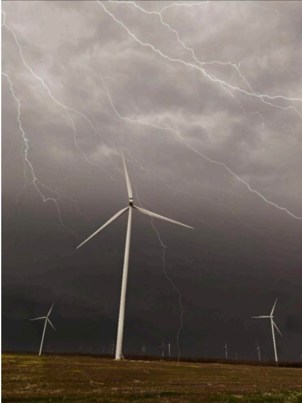
Turbines during lightning event
