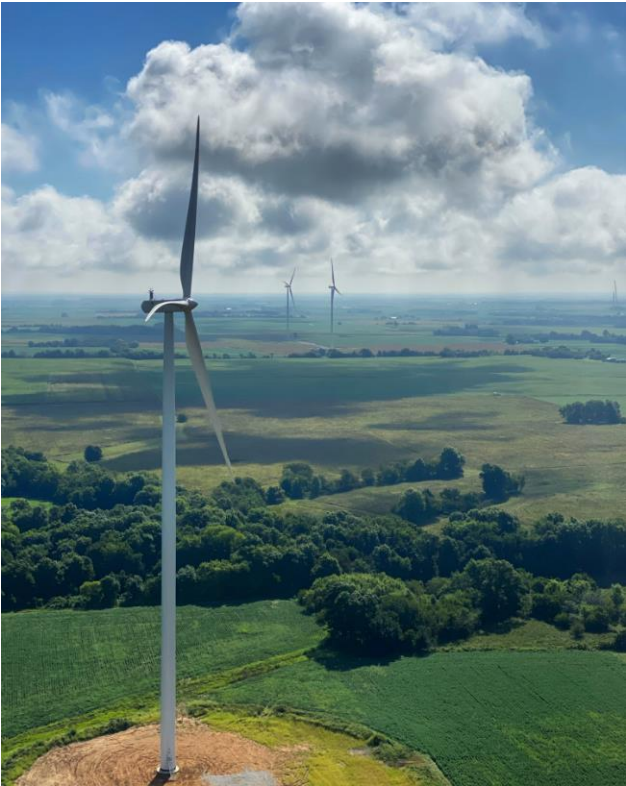
PHOTO 1: UP TOWER PHOTOS
