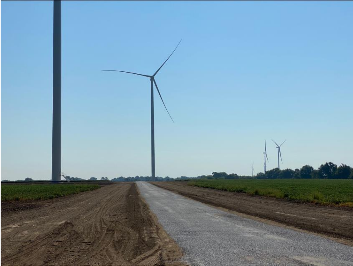
PHOTO 4: FINAL 2" CAP ON T-62/68 ACCESS ROAD
