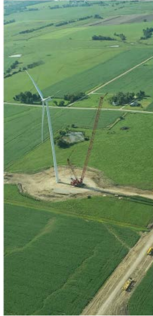
Picture 1. Aerial photography of main erection crane and completed turbine.
