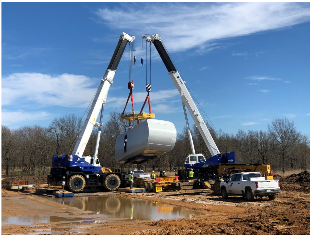
Picture 4. Offloading a V120 nacelle.
