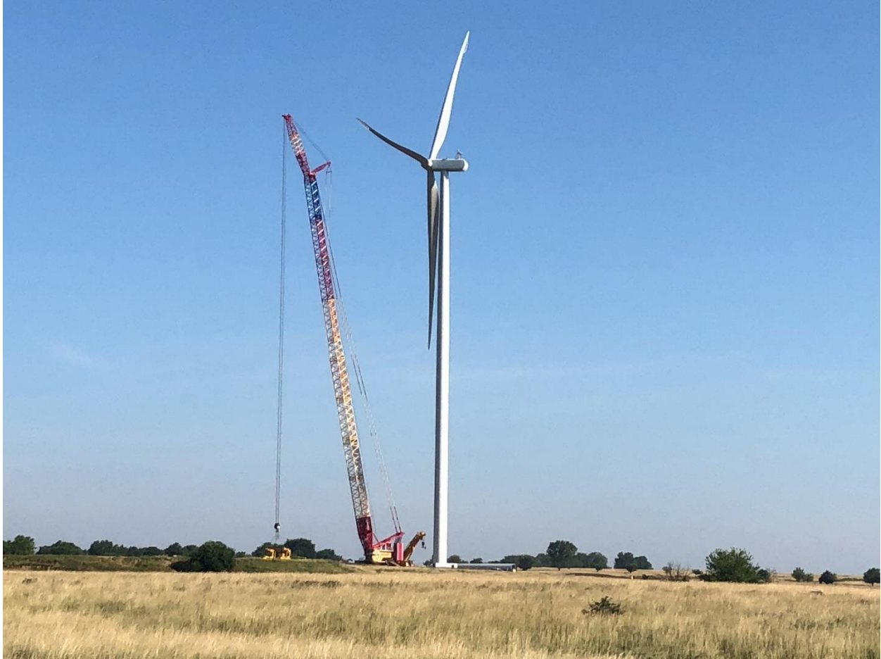
Fully Erected Turbine
