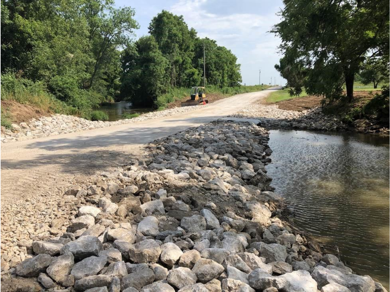
Low Water Crossing on Irving Road - Civil Work
