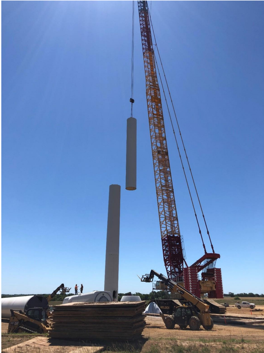
Tower Section Install
