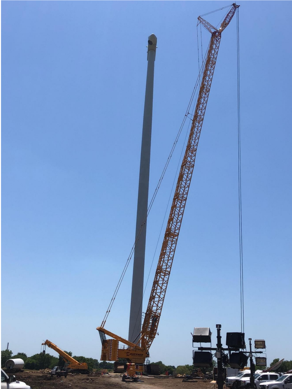
Erected Turbine Prior to Blade Install
