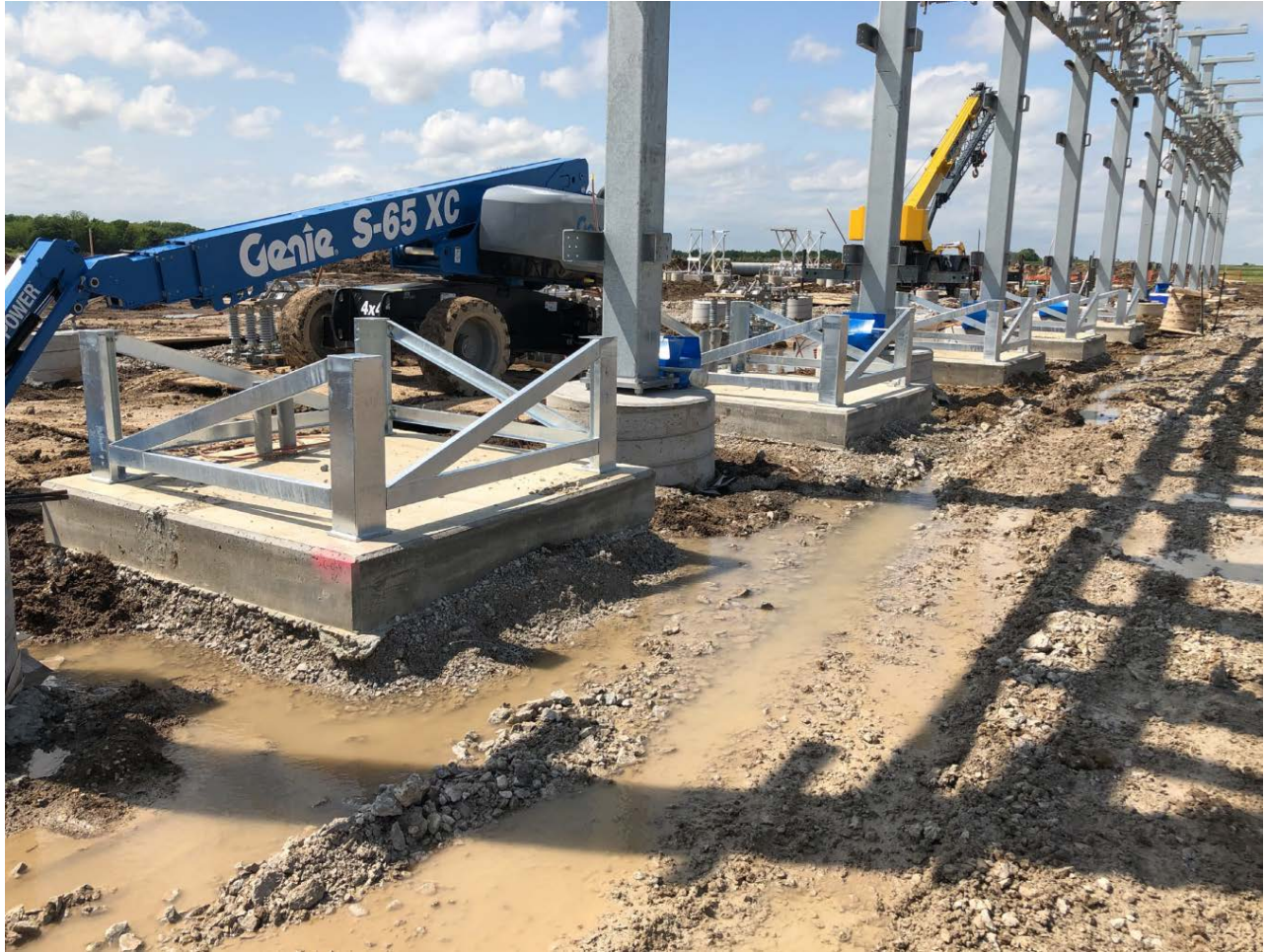
Substation Foundations
