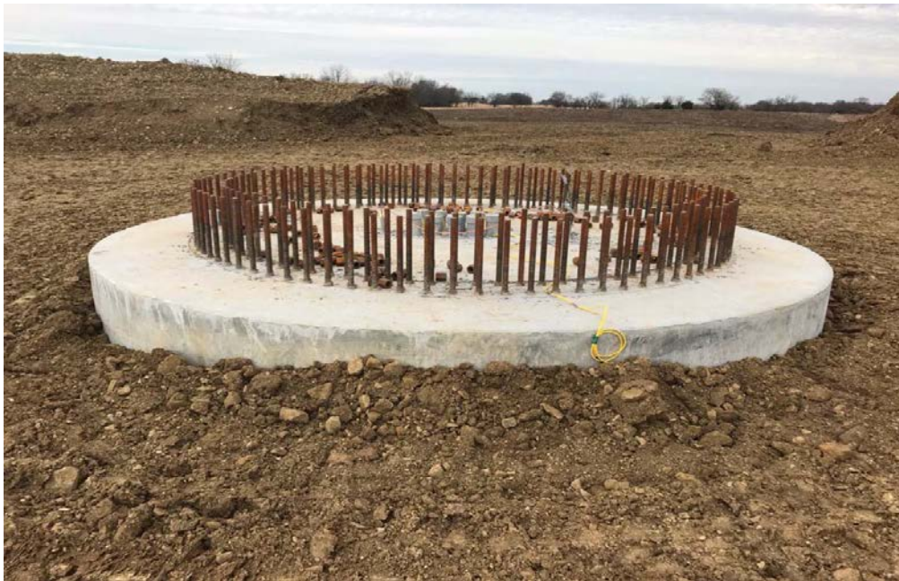
A finished foundation awaits backfill
