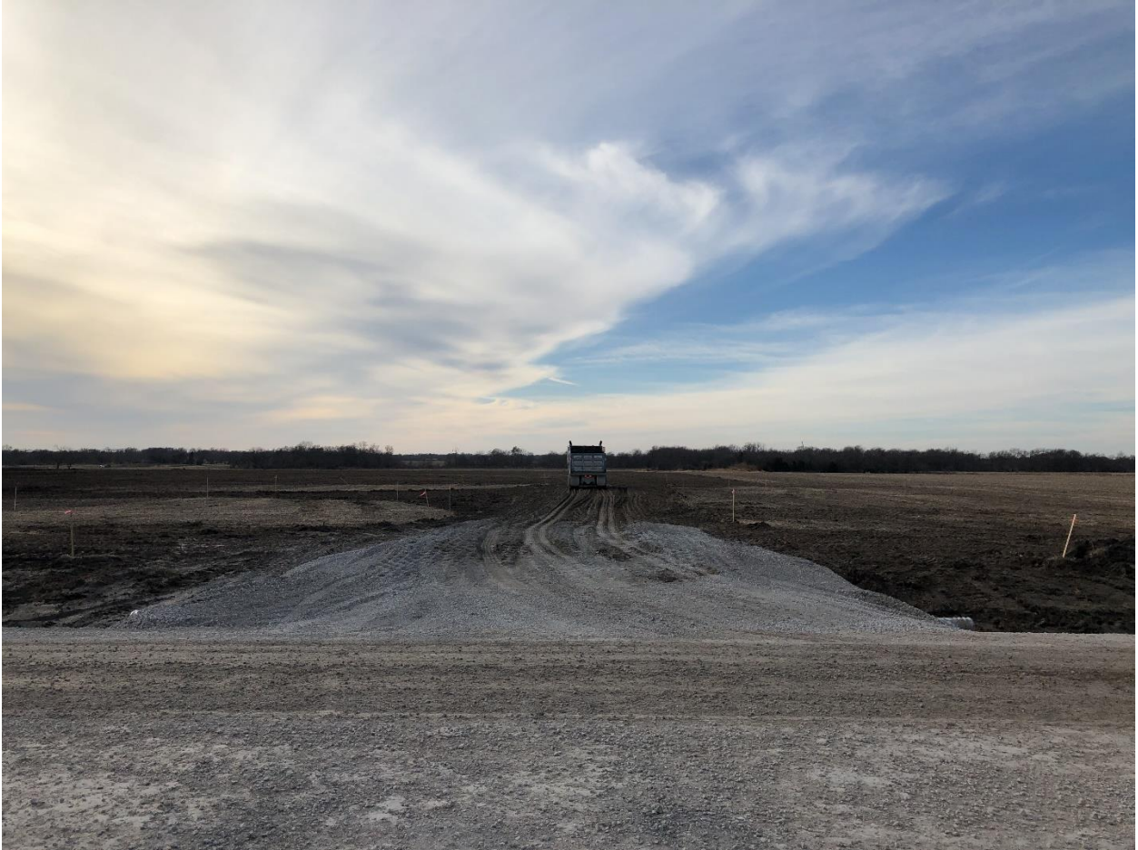
Access road installation to substation
