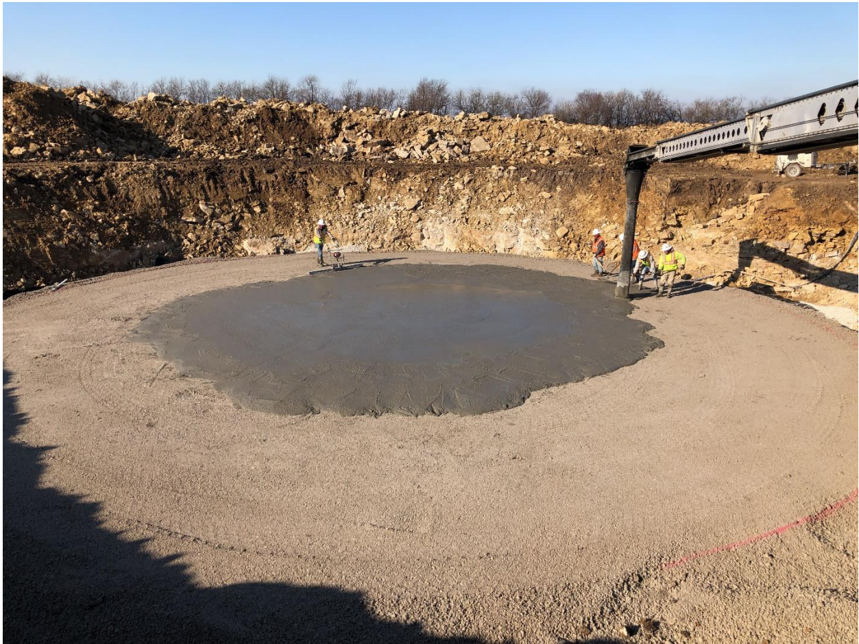
Mudmat being poured for a foundation
