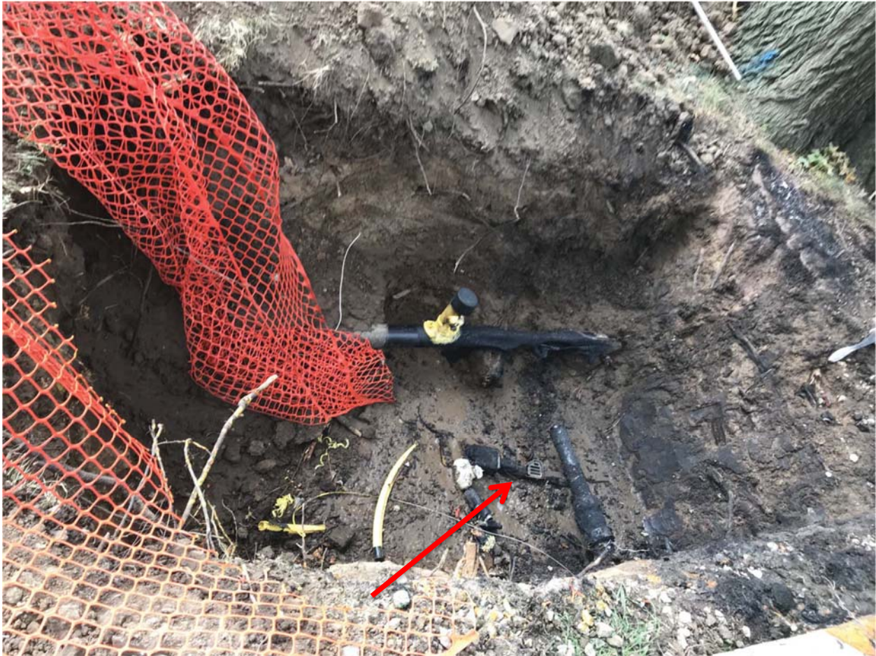
Photograph 1: Photograph looking down into the excavation following the incident. (Source of Photograph: Spire in Response to Staff Data Request 0032). The red arrow (added by Staff) points to electric reciprocating saw shown in Photograph 2. Note: In response to Staff Data Request 0061, Spire answered that the electric reciprocating saw in Photograph 2 is the same electric reciprocating saw at the bottom center of Photograph 1.
