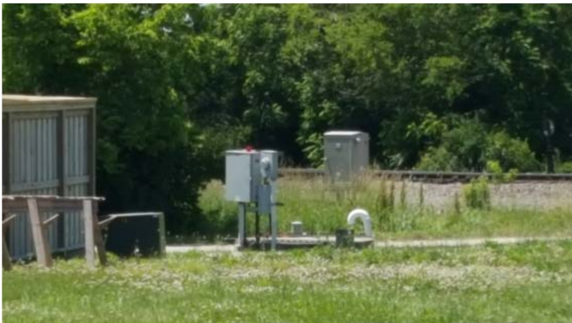
A View of the North West Terrace Lift Station Looking Northwest
