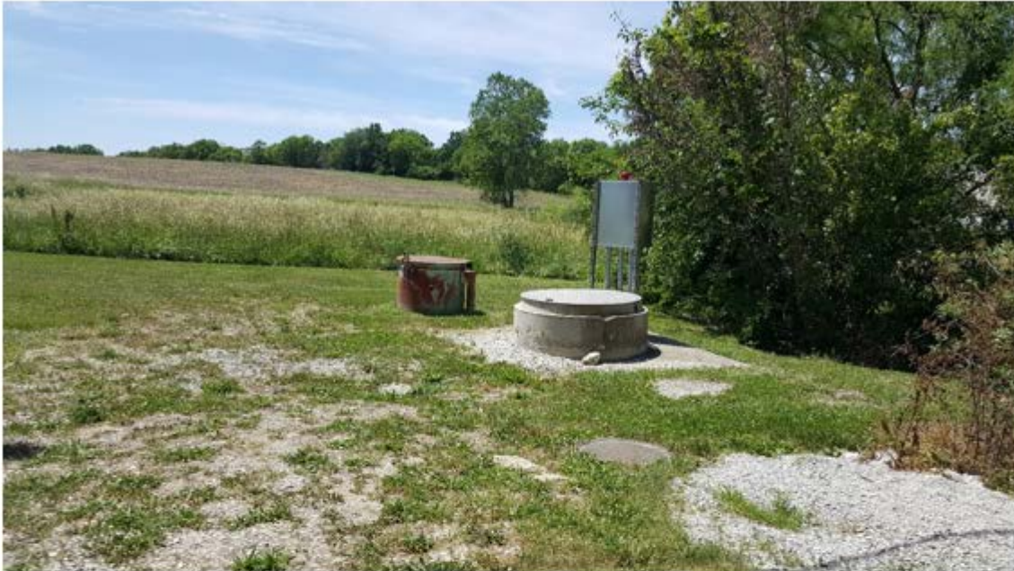
A View of the Raum Lift Station Looking Northwest
