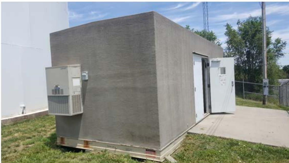
Italian Way Duplex Pumping Station Building Looking Northeast
