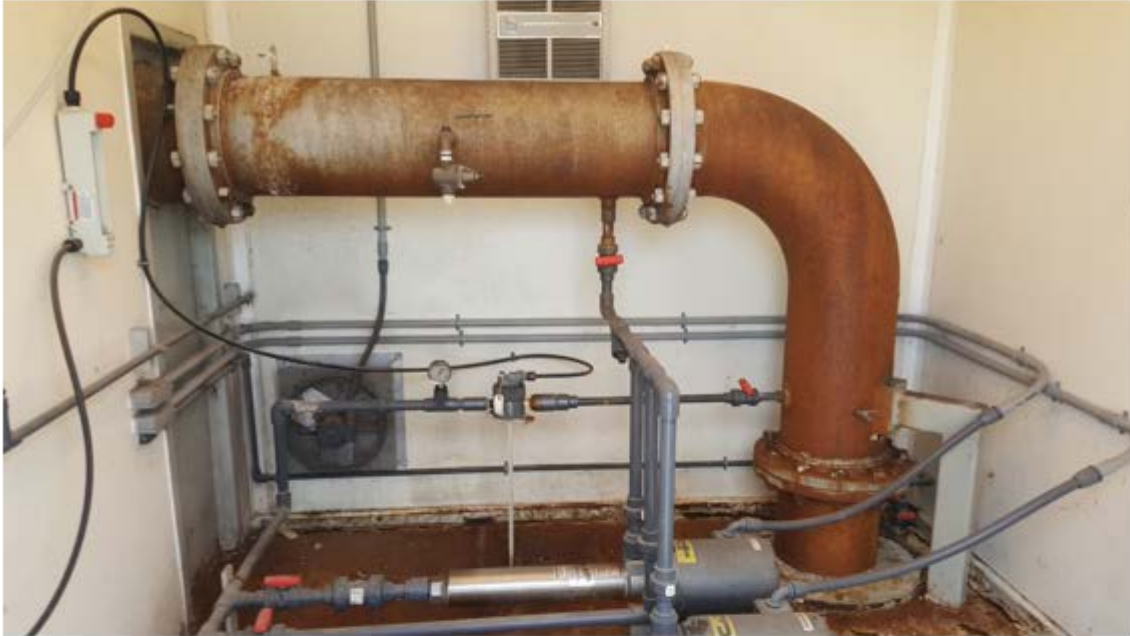
Interior View of the Italian Way Pump Station Building Easternmost Room
