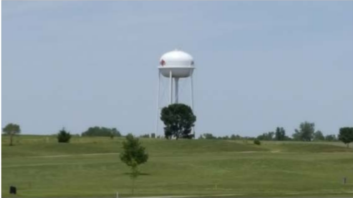
Water Tower West of Golf Course Looking North
