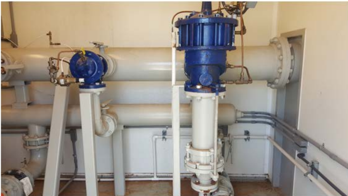
Interior View of the Italian Way Pump Station Building Westernmost Room
