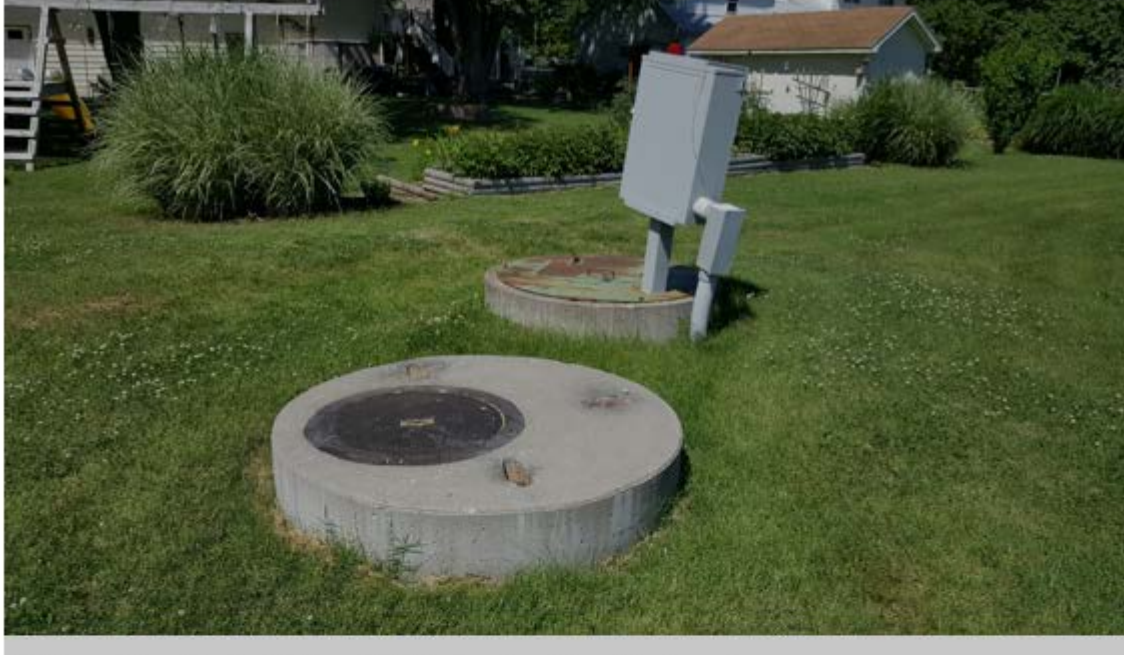
A View of the Musket Drive Lift Station Looking Northeast
