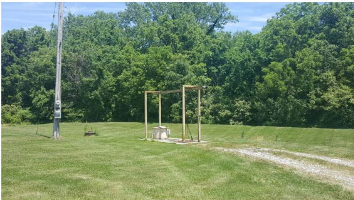
A View of the Lagoon Lift Station Looking East
