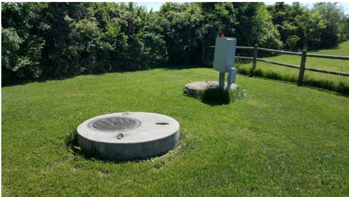
A View of the Powderhorn Drive Lift Station Looking Southwest
