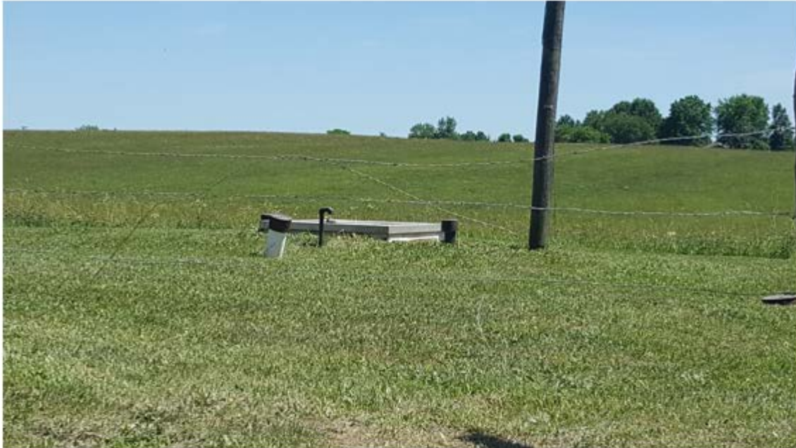
A View of the Vibbard Pump Station Looking Southeast
