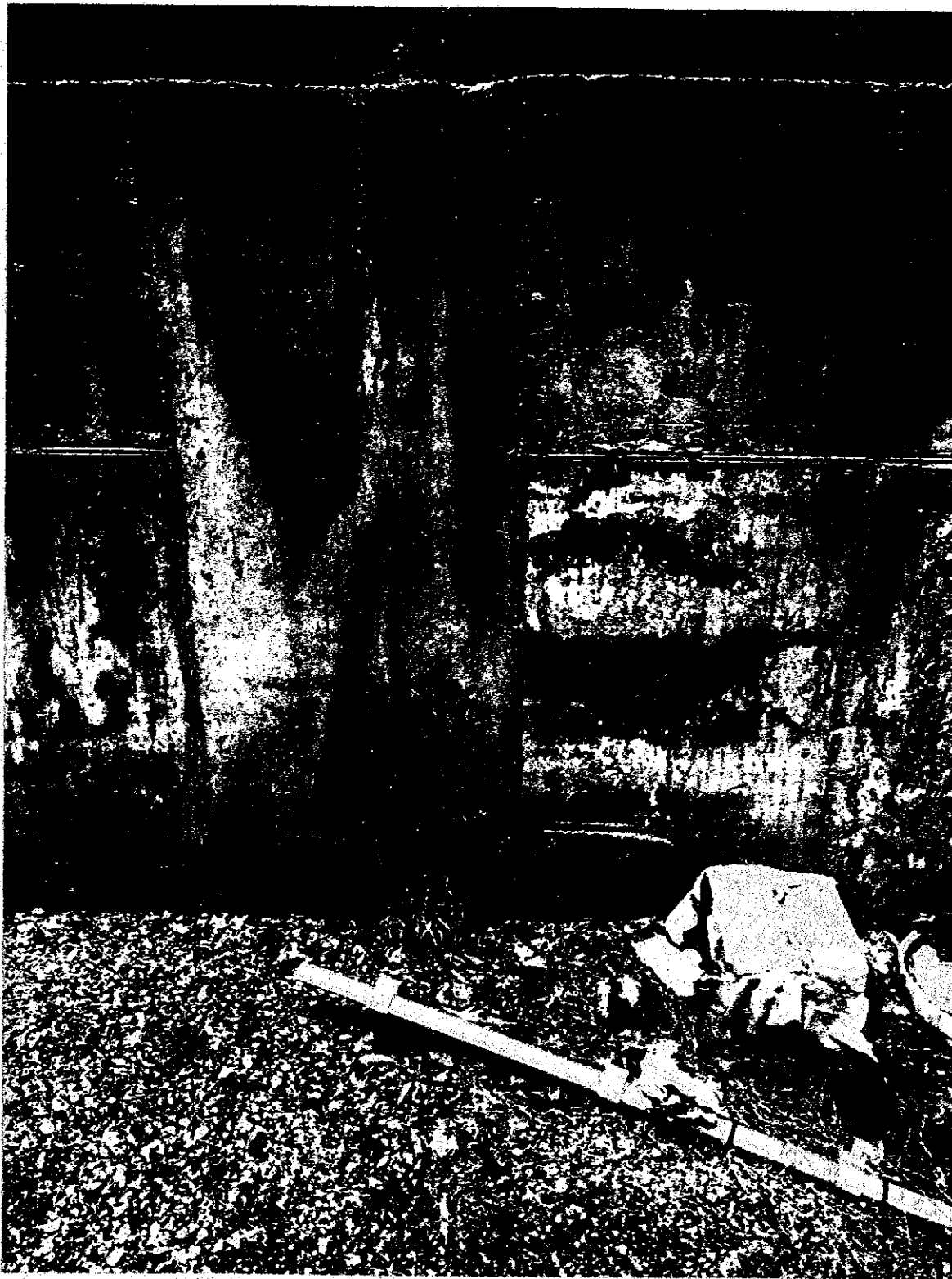
Figure 15-Sand Filter Bed Crack was Leaking During January 30, 2016 Visit
