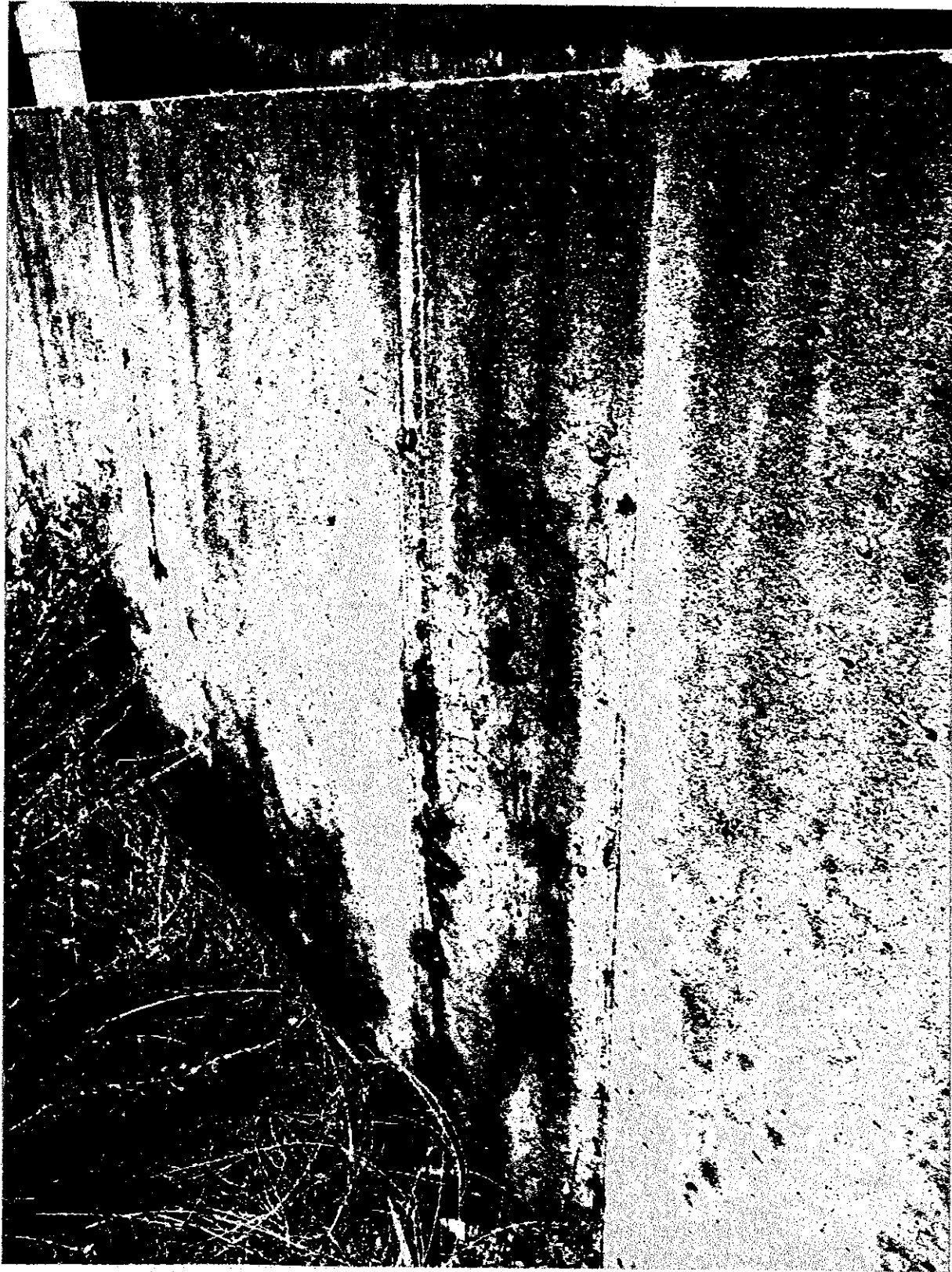
Figure 2-Sand Filter Bed Crack was Leaking During January 30, 2016 Visit
