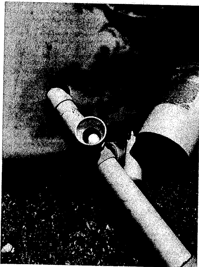
Figure 23-Homemade Chlorinator
