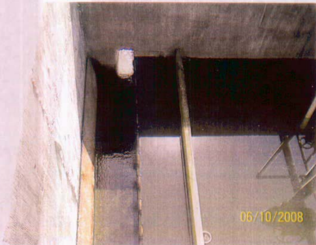
View of Clarifier Weir
