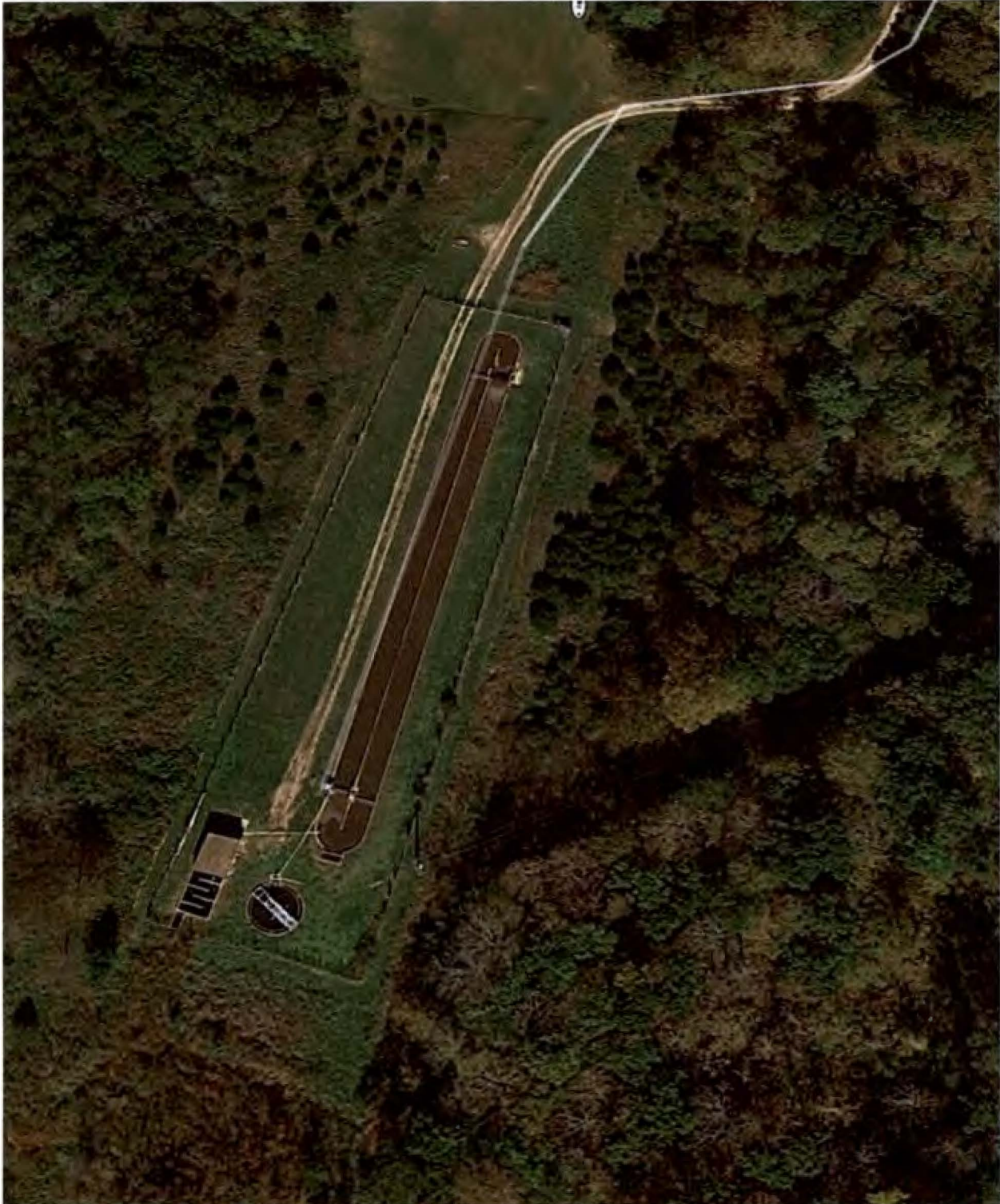
Aerial view of Terre Du Lac Oxidation Ditch via Google Earth
