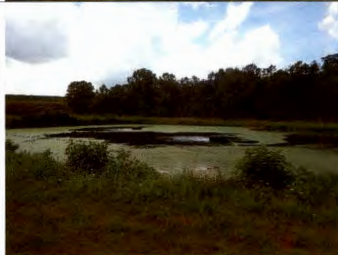
Photograph #: 003 Taken by: Wesley Hargraves Entity: Terre Du Lac North - Three Cell Lagoon Permit: MO0035700 Location: St. Francois County Description: View of secondary cell. Taken facing southwest. Date Taken: July 10, 2019 Program: WPC Unit
