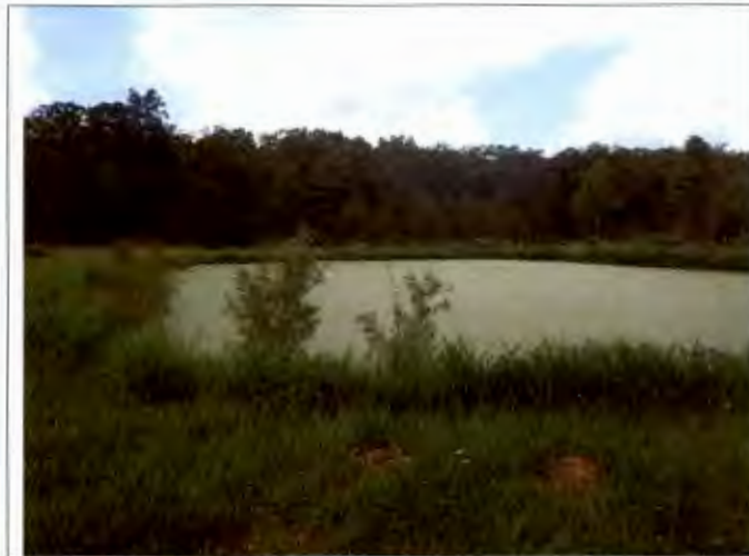
Photograph #: 004 Taken by: Wesley Hargraves Entity: Terre Du Lac North - Three Cell Lagoon Permit: MO0035700 Location: St. Francois County Description: View of third cell. Taken facing west. Date Taken: July 10, 2019 Program: WPC Unit
