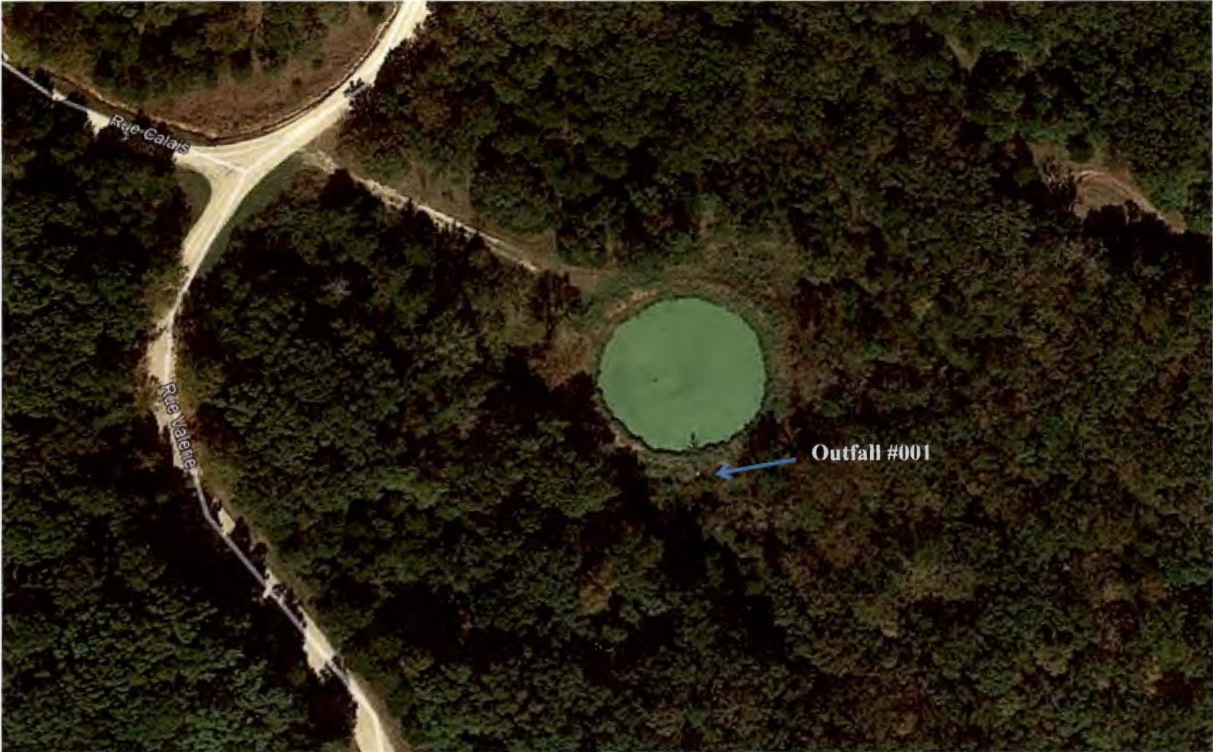
Aerial view of Terre Du Lac South - One Cell Lagoon via Google Earth
