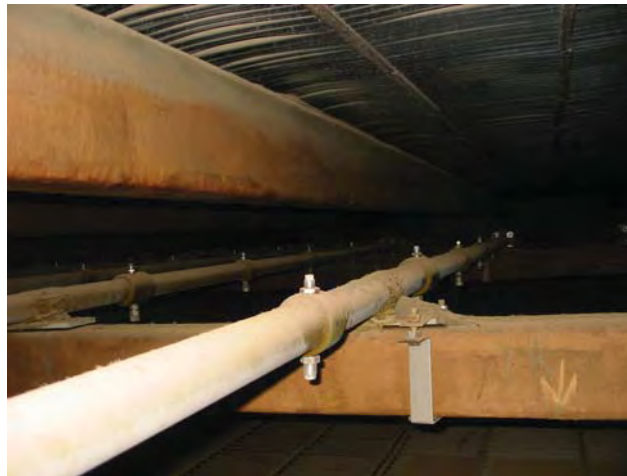
Figure 2-5 – Between-Stage Mist Eliminator Wash Nozzles
