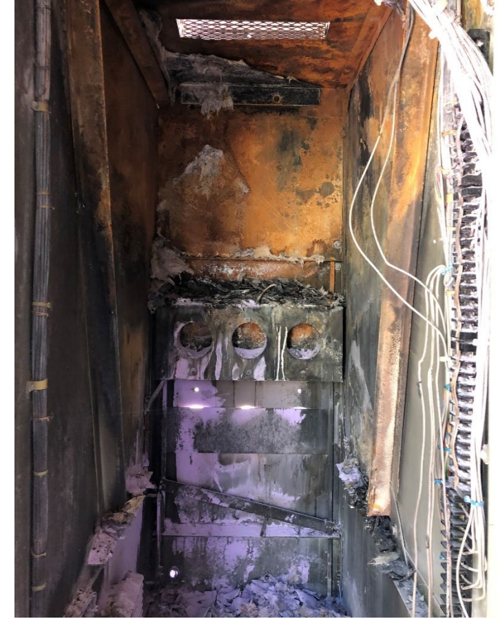
Switchgear Failure (Mullanphy)
