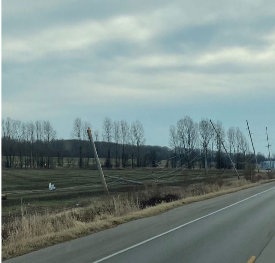
Non-Hardened Line, Cascading Failure
