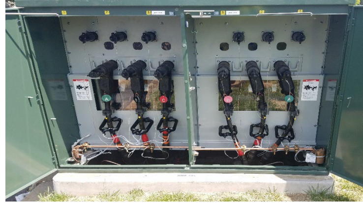
New Automated Switchgear
