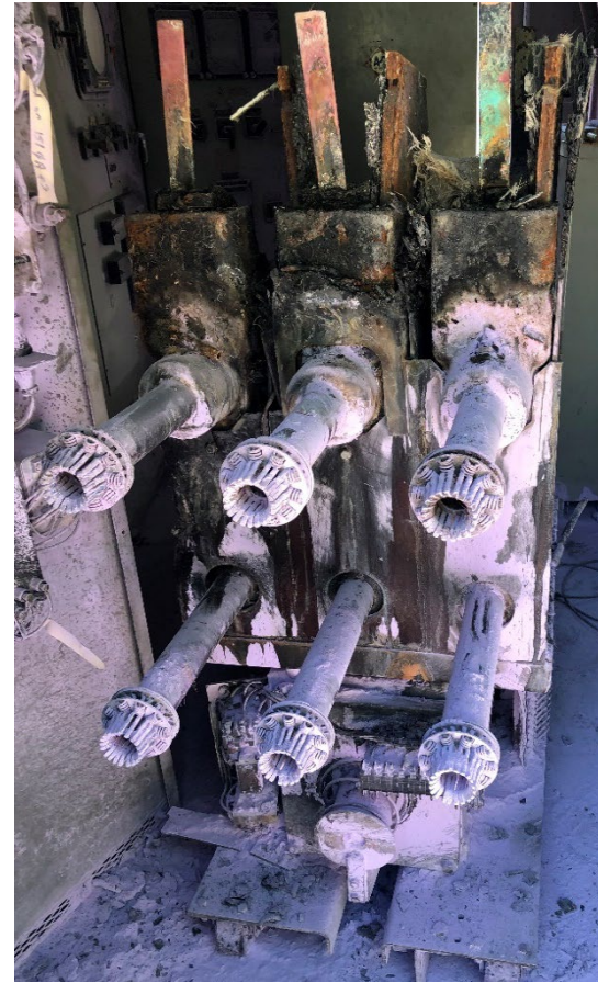
Switchgear Failure (Mullanphy)
