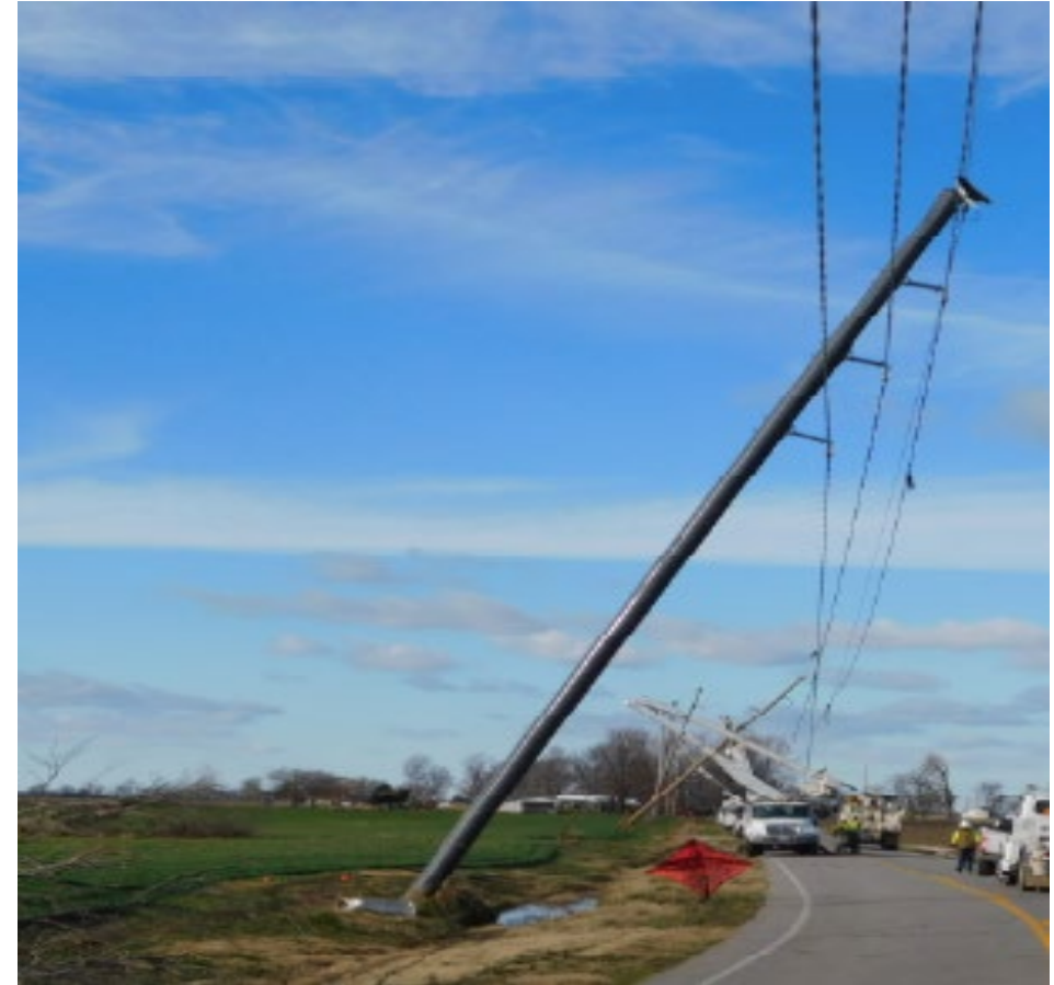
Hardened Line, Limited Cascading Failure
