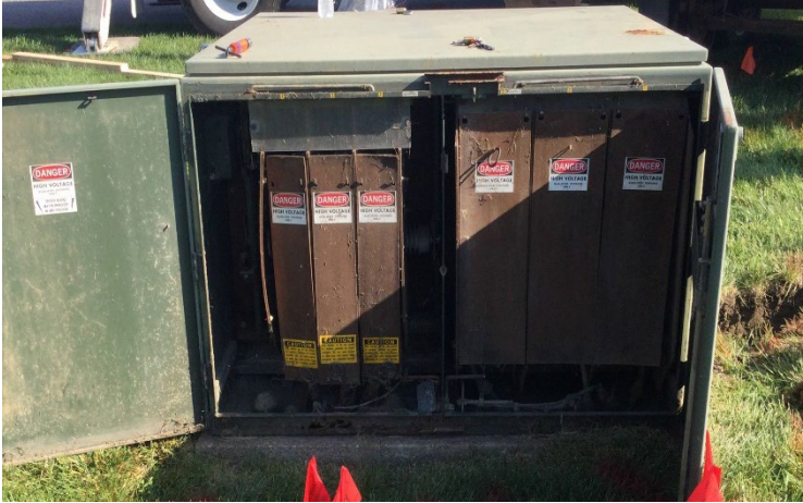
Manual Switchgear Before Replacement
