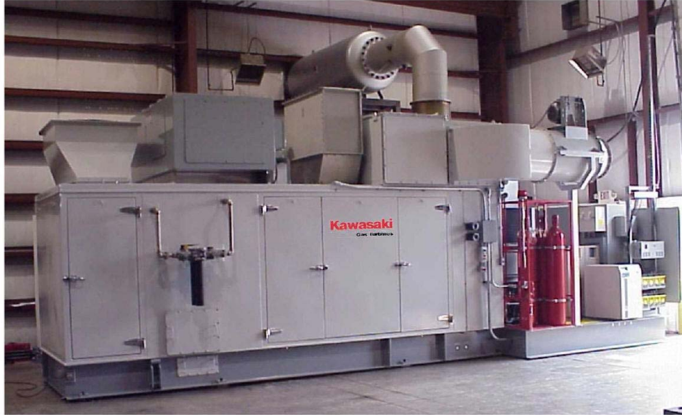
Figure 3-2 Kawasaki GPB151X Gas Turbine Installation
