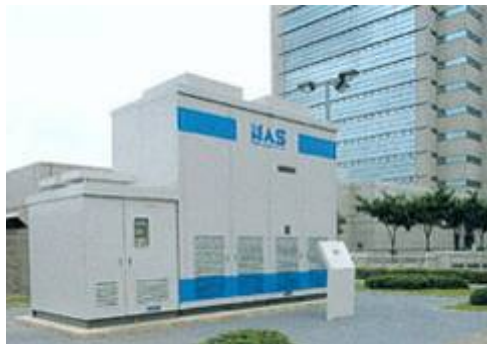
Figure 3-12 NaS Peak Shaving Battery System 5
