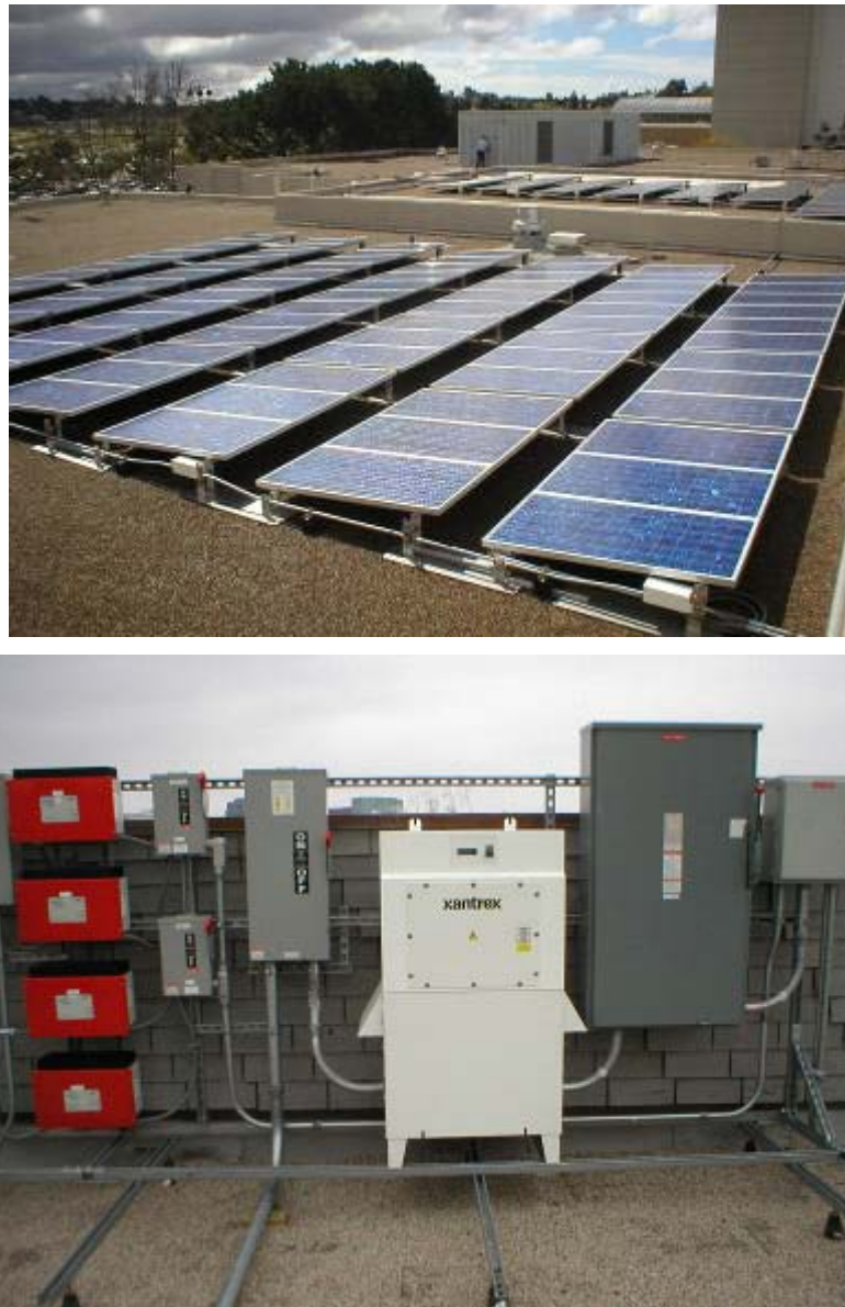
Figure 3-8 PV Array and Inverters
