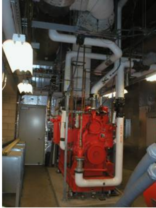
Figure 3-1 Waukesha VGF18GSID (280 kW) Reciprocating Engine CHP
