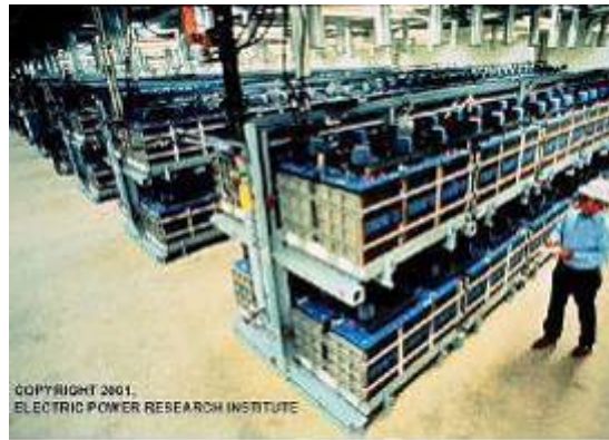
Figure 3-11 Utility Scale Battery Energy Storage System
