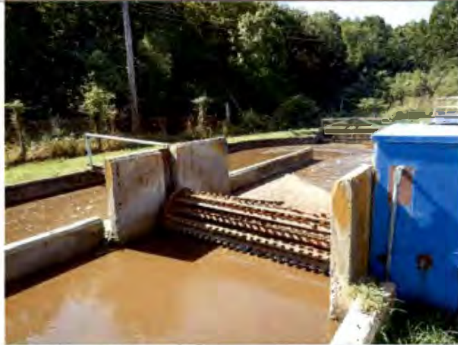
Photograph #: 002 Taken by: Wesley Hargraves Entity: Terre Du Lac Oxidation Ditch Permit: MO0095311 Location: St. Francois County Description: View of southern rotor. This rotor was not operable at the time of the inspection. Taken facing south. Date Taken: July 10, 2019 Program: WPC Unit
