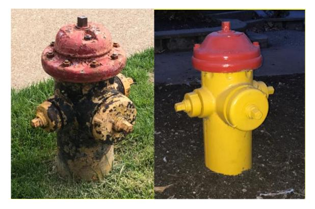
As I explain in my direct testimony, if painting is not done consistently, hydrants can develop surface corrosion that not only looks bad, but can lead to performance problems in the long term. The Company is seeking a level of hydrant painting expense that supports a more cost effective level of service for our customers over the long term.
