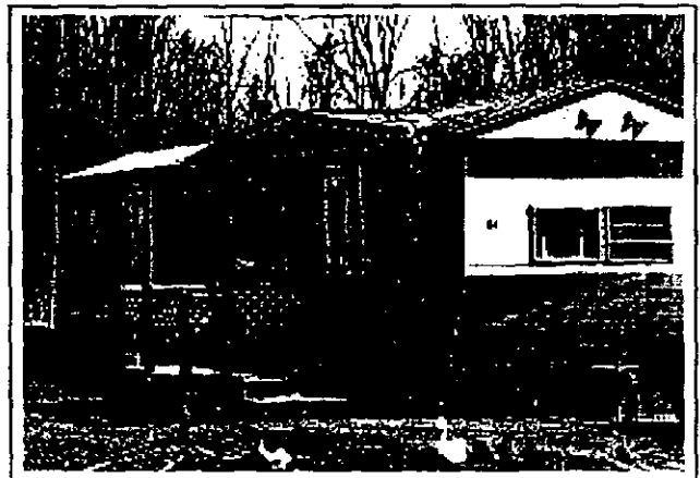
Skirting under a mobile home is not as important for the heating bill as belly board insulation, which can be blown in by weatherization crews.
