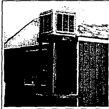
Evaporative chillers (swamp coolers) often mean large leaks.
