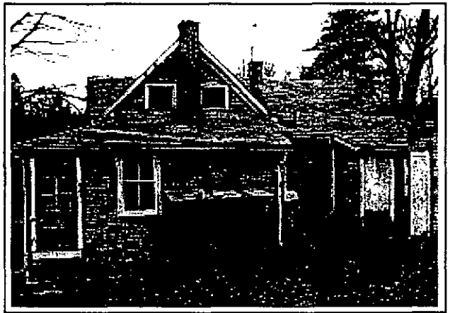
Built in sections over many years, this dwelling has major leaks between the main house and newer additions.
