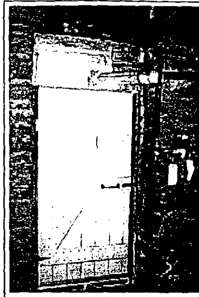
A new bulkhead door and insulated sheathing isolate the area under a porch, thus solving a major infiltration problem.
