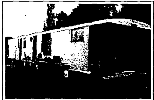
Mobile homes with poor foundations often develop major structural problems.
