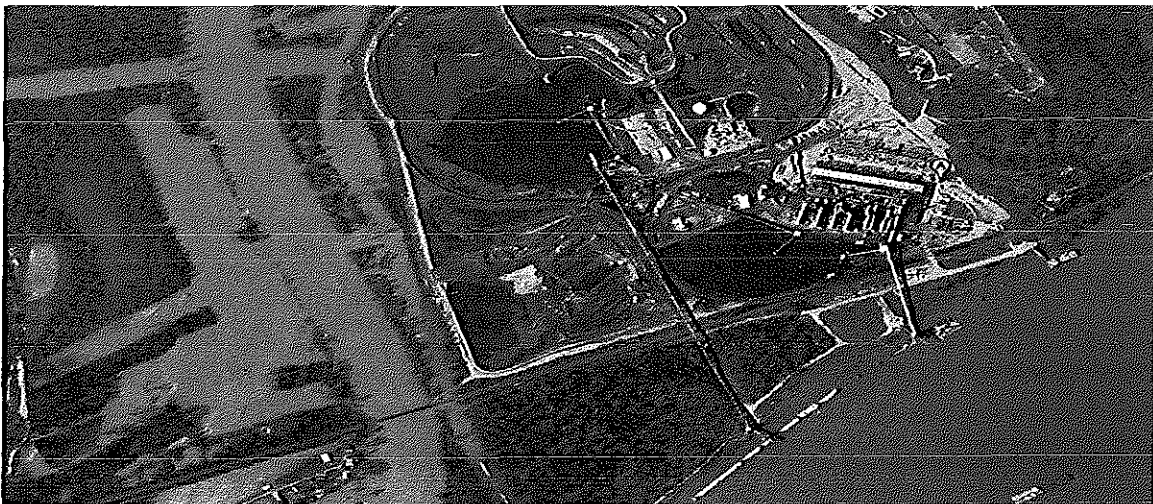
Ameren UE Meramec Power Plant in St. Louis County (Google Satellite Map)
