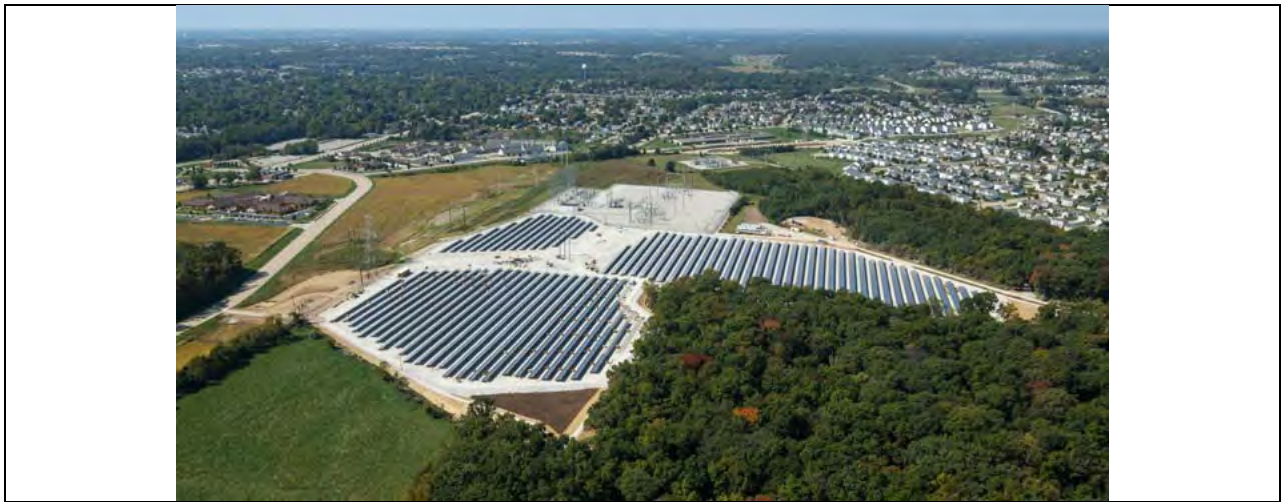
10 Figure 12. Ameren MO 5.7 MW O’Fallon Renewable Energy Center, Operational in 11 December 2014 82
