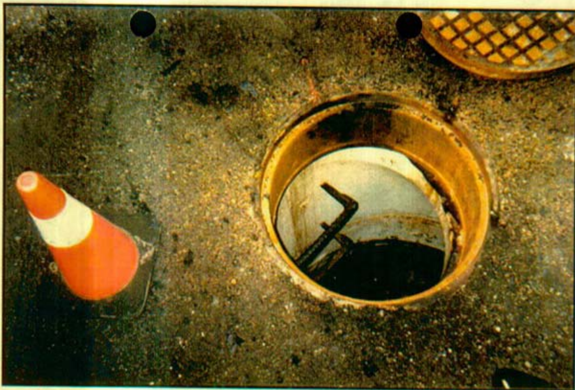
Photograph 1: View of the communications vault where the natural gas ignition and flash fire occurred. Note the dark discoloration around the upper portion of the vault. (Photograph provided by MGE.)
