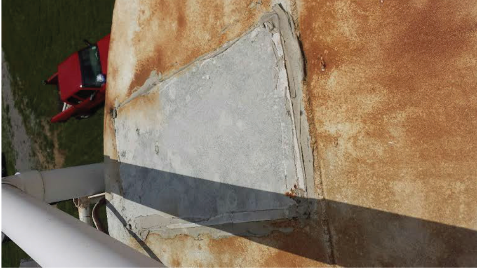
Temp Patch Top of Tank
