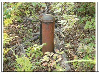
PHOTOGRAPH# 4 TAKEN BY: Darrell Barber ENTITY: Reflections Condos PERMIT: MO3071337 LOCATION: Southeast of well house DESCRIPTION: Abandoned well approximately 135 feet from the public water system well for Reflections Condos. The abandoned well is not located on property owned by Great Southern Bank or Reflections Condominium Owners Association, Inc. DATE TAKEN: August 9, 2017 PROGRAM: Public Drinking Water Branch Kathleen Spero Abandoned Well Report August 9, 2017
