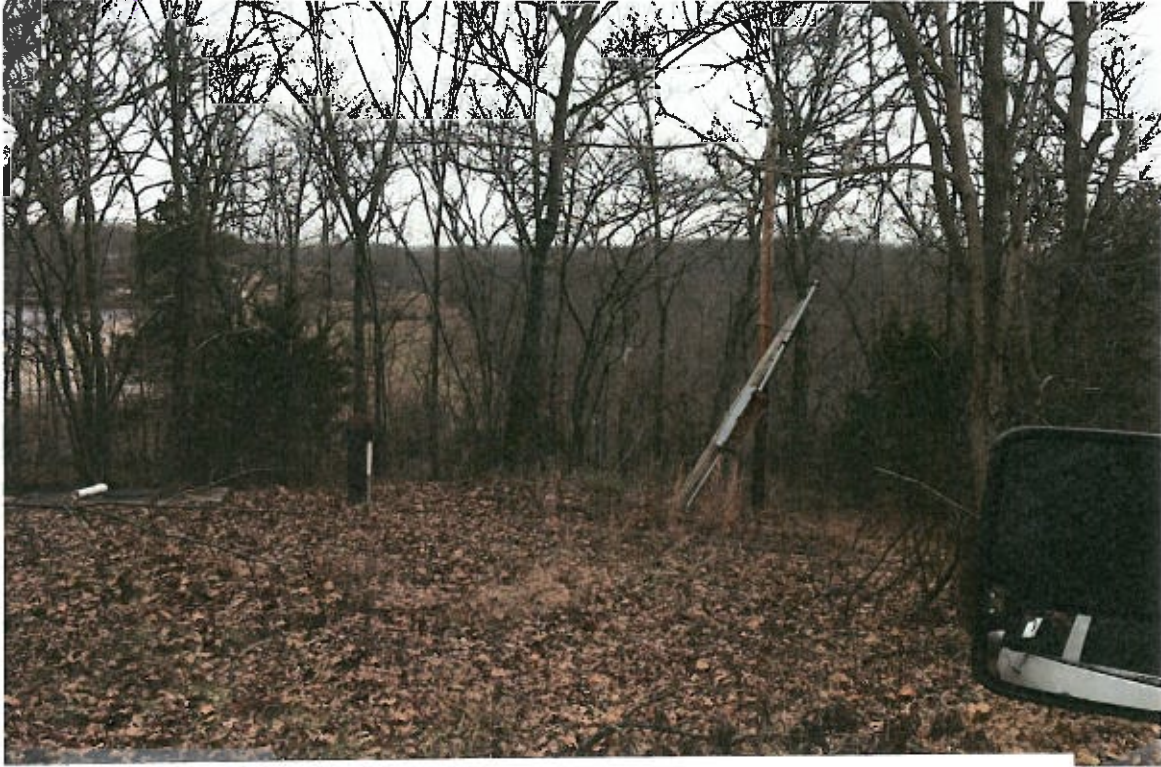
Well #2 open Well Head
