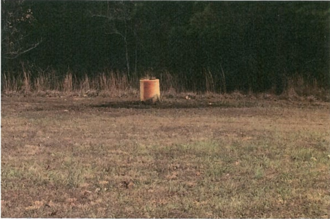
Irrigation head for Wastewater Disposal (typical)
