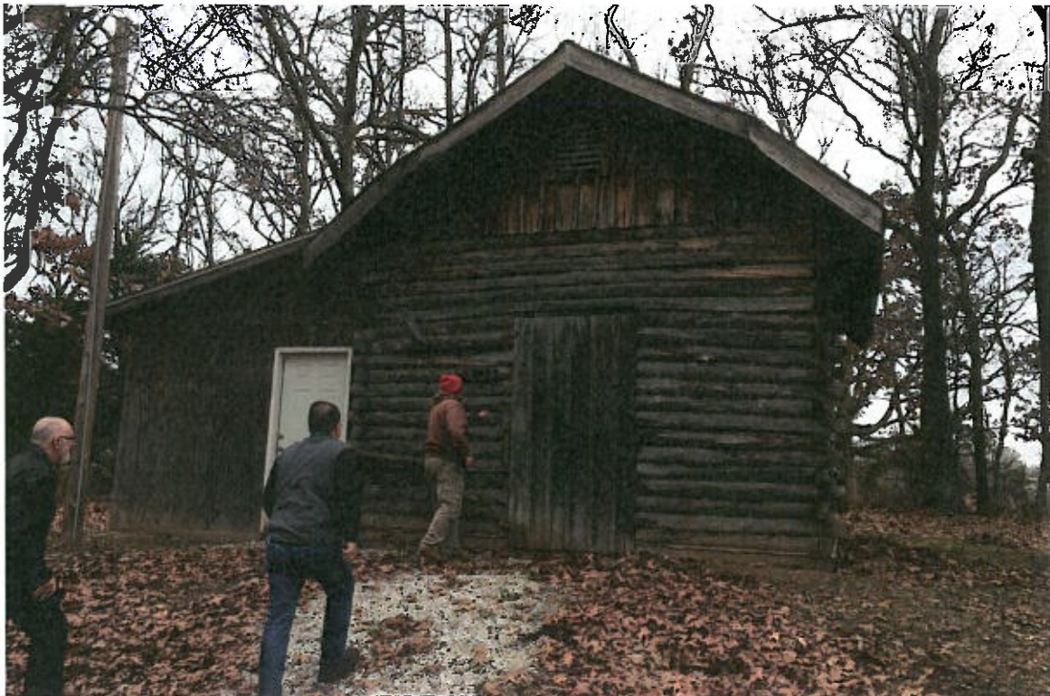
Well #1 Well House
