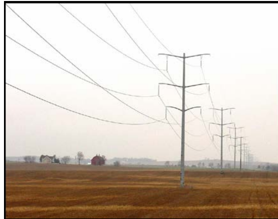
Figure 2 Typical Single-Pole, Double-Circuit Structure
