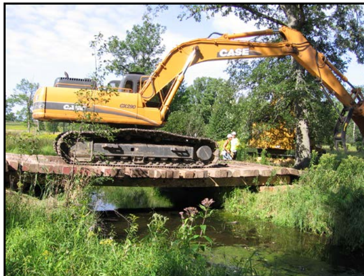
Figure 5 Temporary Bridge Structure Spanning a Waterway
