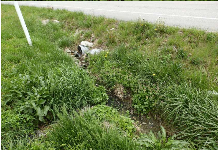
Photograph #: 5 Taken by: Michael Heaton Entity: BCRSD, Lee Heights Wastewater Treatment Facility Permit: #MO-0102113 Location: Boone County Description: Flow from the outfall flows to the roadside ditch and through the culvert. Date Taken: May 2, 2018 Program: WPC Unit
