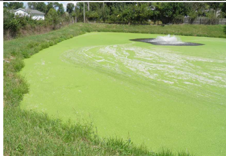
Photograph #: 5 Taken by: Michael Womack Entity: BCRSD - Highfield Acres Wastewater Treatment Facility Permit: #MO-0053376 Location: Boone Description: Observation of Outfall #002 lagoon cell. Duckweed is observed within the lagoon and erosion damage is observed at the southwest inner lagoon berm of the lagoon (bottom left corner). The aerator appears to be operating properly. Date Taken: September 1, 2016 Program: WPC Unit
