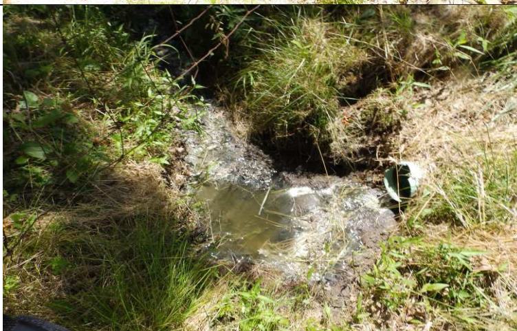
Photograph #: 6 Taken by: Leland Maize Entity: BCSD, Cedar Gate Subdivision Permit: #MO-0096415 Location: Boone County Description: Outfall pipe with a white film in the area directly below the outfall pipe. Date Taken: June 7, 2016 Program: WPC Unit
