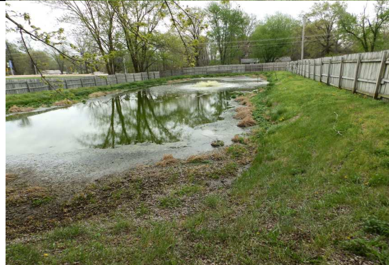
Photograph #: 2 Taken by: Michael Heaton Entity: BCRSD, Lee Heights Wastewater Treatment Facility Permit: #MO-0102113 Location: Boone County Description: Overview of the lagoon. Aerator was operational in the lagoon. Date Taken: May 2, 2018 Program: WPC Unit
