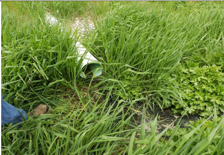
Photograph #: 4 Taken by: Michael Heaton Entity: BCRSD, Lee Heights Wastewater Treatment Facility Permit: #MO-0102113 Location: Boone County Description: Outfall #001. Outfall was not discharging at the time of the inspection. Date Taken: May 2, 2018 Program: WPC Unit
