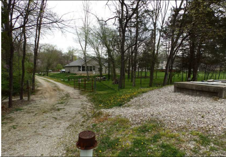
Photograph #: 1 Taken by: Michael Heaton Entity: BCRSD, Oberlin Valley Wastewater Treatment Facility Permit: #MO-0117323 Location: Boone County Description: Front entrance to the facility. Gate to facility with an all-weather access road. Date Taken: May 2, 2018 Program: WPC Unit
