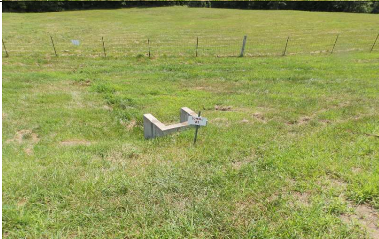
Photograph #: 6 Taken by: Leland Maize Entity: BCRSD, Quarter Mile Hills Subdivision Permit: #MO-0126446 Location: Boone County Description: Location of the outfall with a sign marking the location. Date Taken: July 27, 2016 Program: WPC Unit
