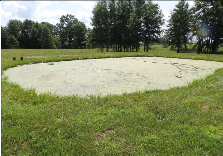
Photograph #: 4 Taken by: Leland Maize Entity: BCRSD, Quarter Mile Hills Subdivision Permit: #MO-0126446 Location: Boone County Description: Tertiary lagoon cell covered with duckweed. Date Taken: July 27, 2016 Program: WPC Unit
