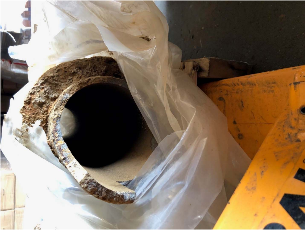
Figure 13, Spire East, Cast Iron
