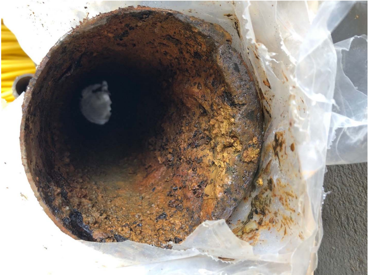
Figure 49, Spire East, Cast Iron
