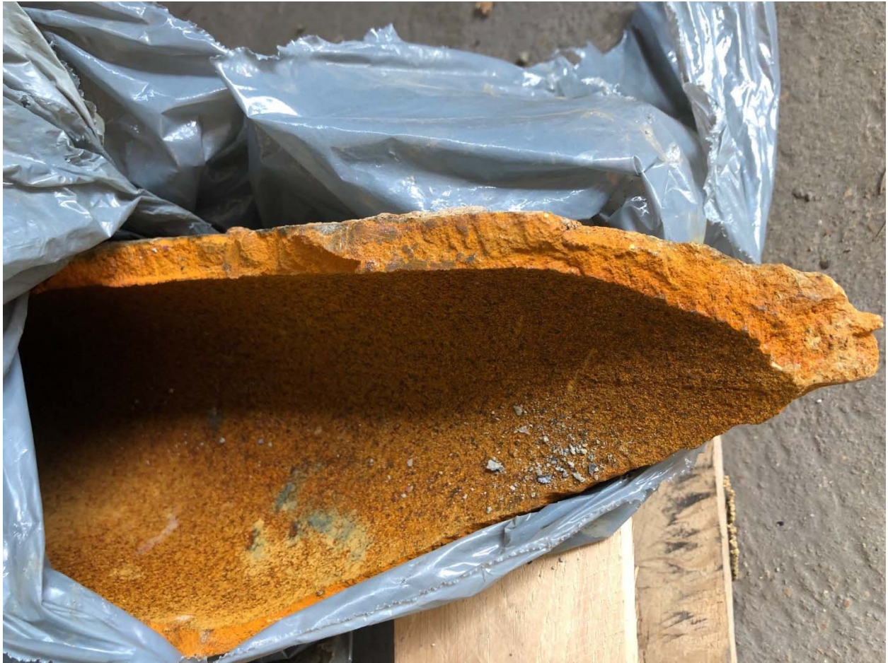
Figure 26, Spire East, Cast Iron
