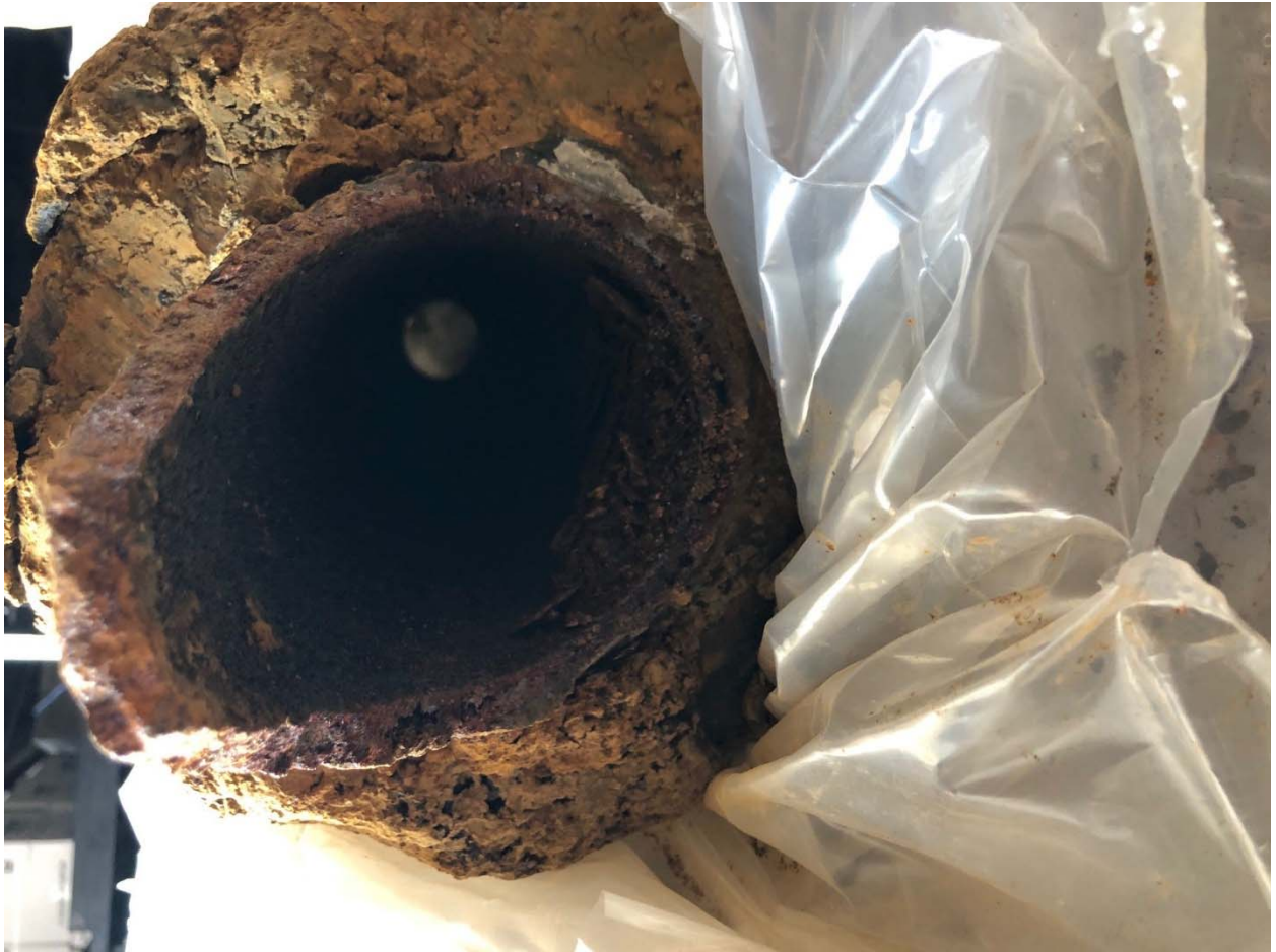
Figure 17, Spire East, Cast Iron
