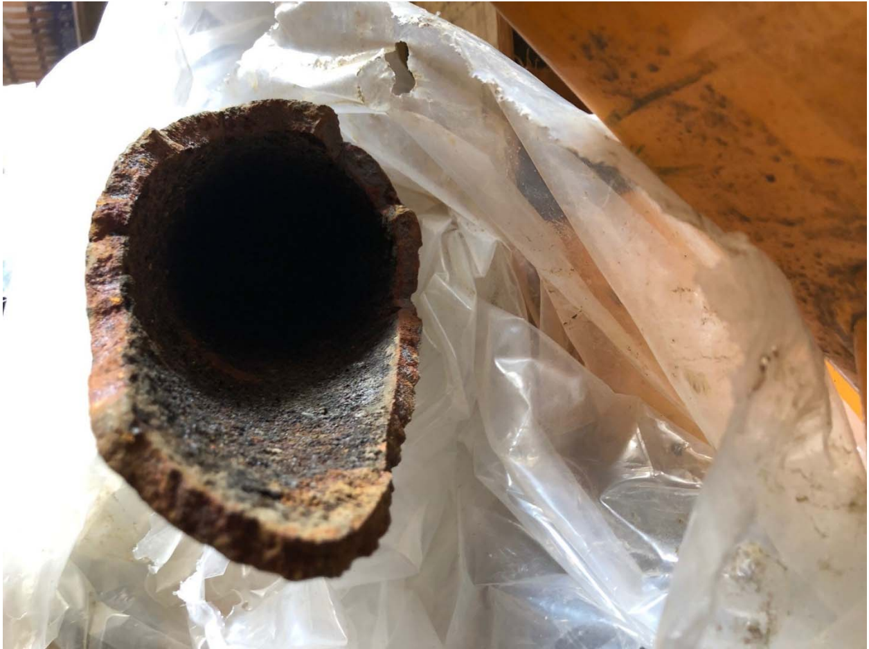
Figure 11, Spire East, Cast Iron
