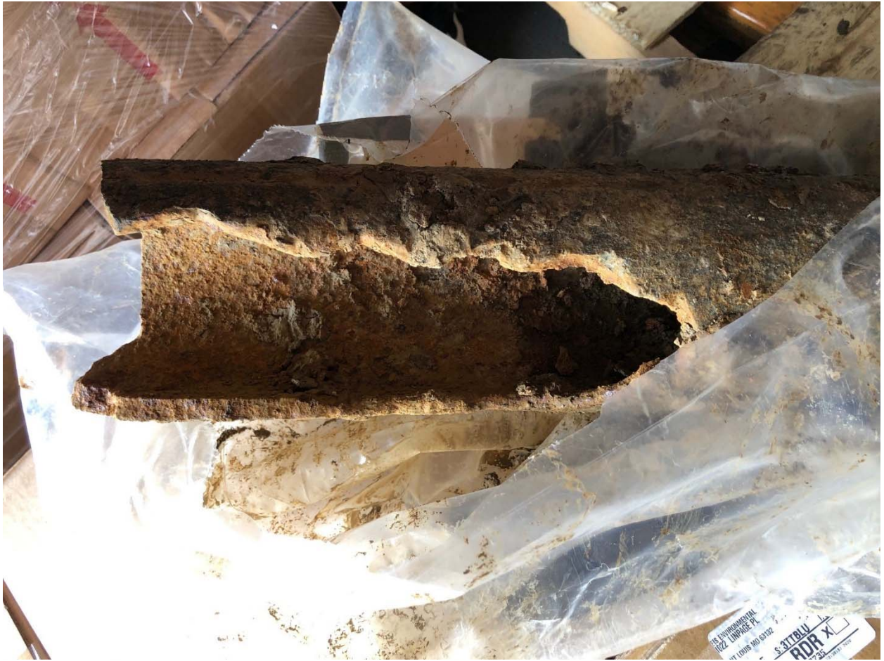
Figure 9, Spire East, Cast Iron
