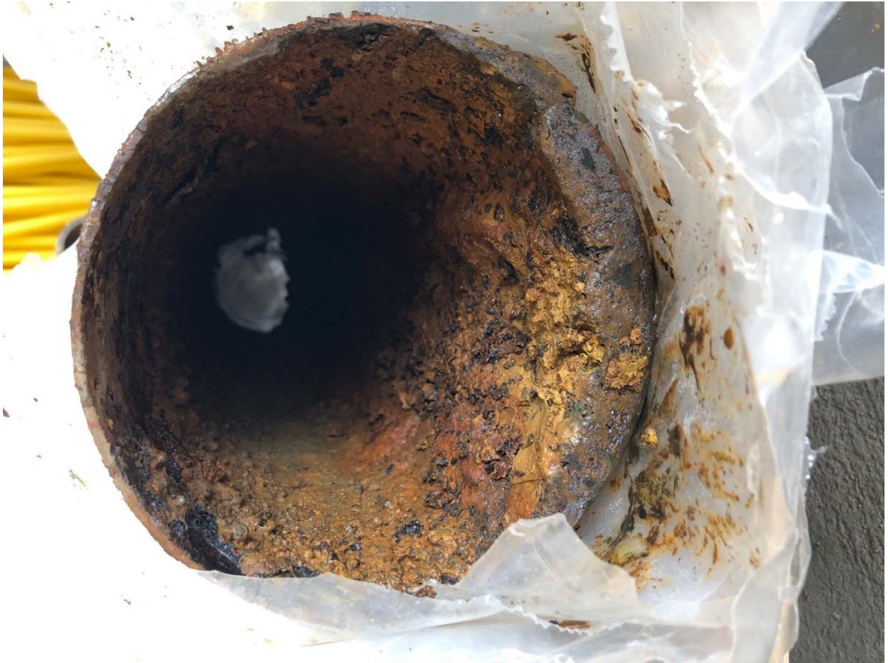
Figure 50, Spire East, Cast Iron
