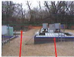
Old WWTP Converted to I&I Storage (you can see it's filled in picture)
