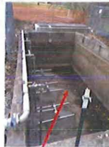
Conversion of Disconnected Concrete Tank to Sludge Holding
