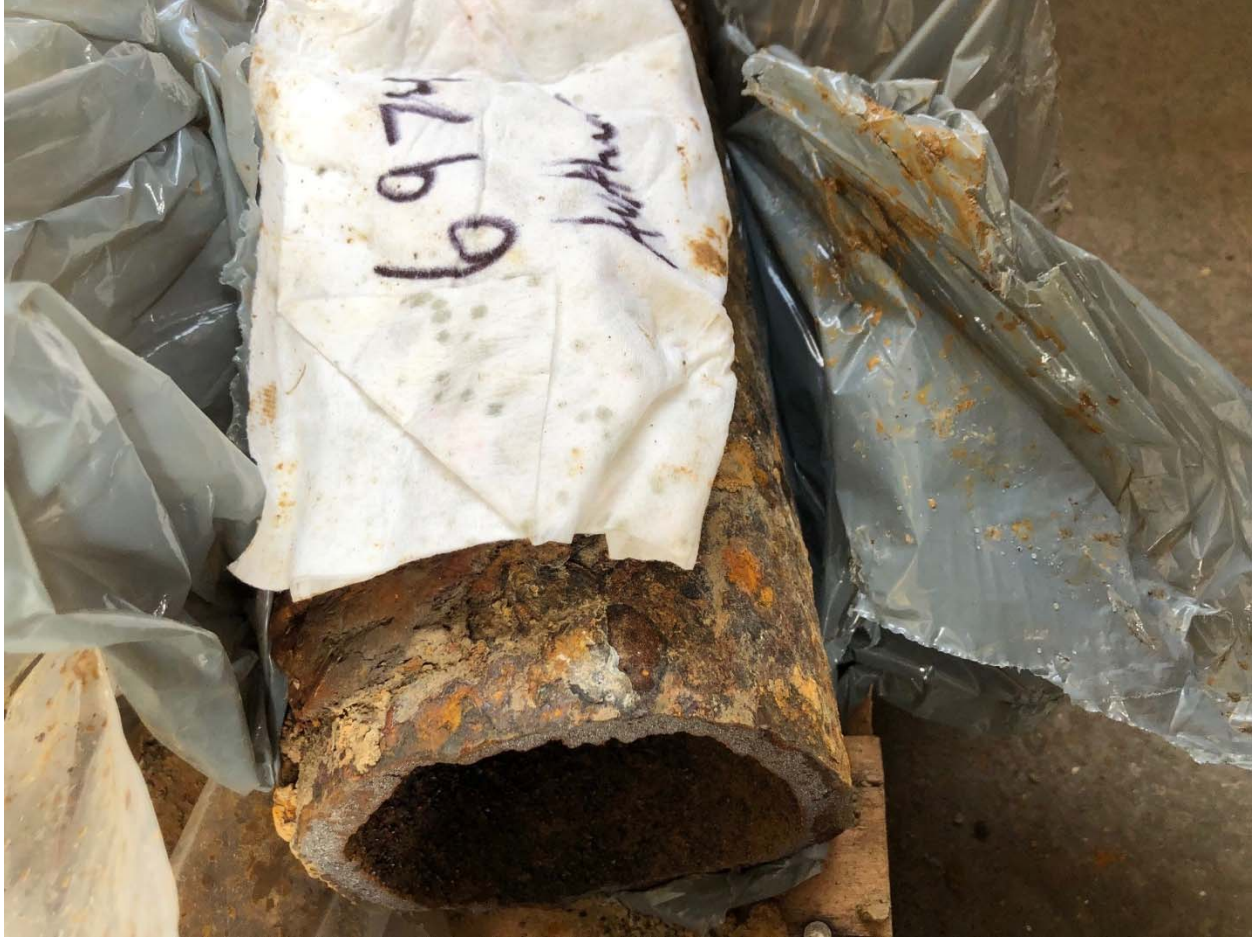
Figure 42, Spire West, Cast Iron
