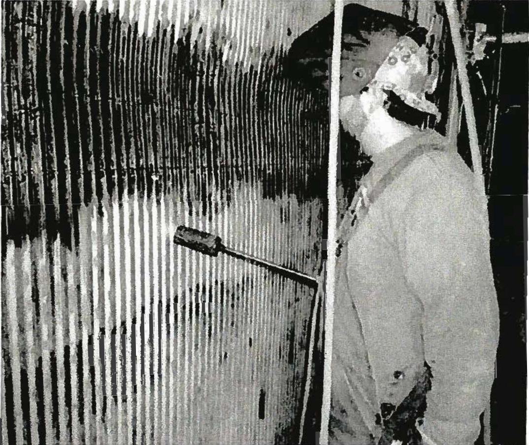
Alstom – Preheating Tube No. 95 on Left Furnace Wall
